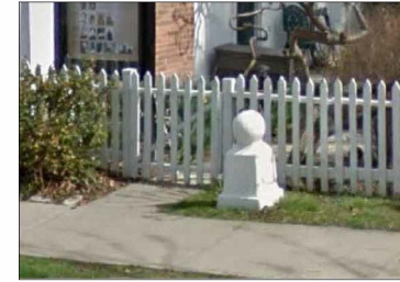
IMAGE OF FENCE TAKEN FROM 156 QUEEN STREET, NIAGARA ON THE LAKE.
