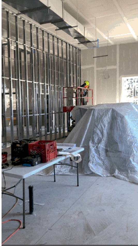
Figure 3: Daycare Addition Construction – Interior wall framing
