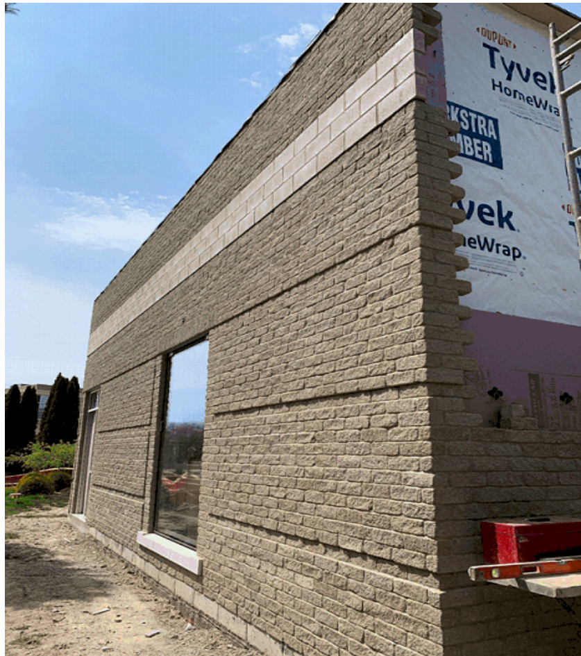
Figure 1: Daycare Addition Construction – Brick Installation
