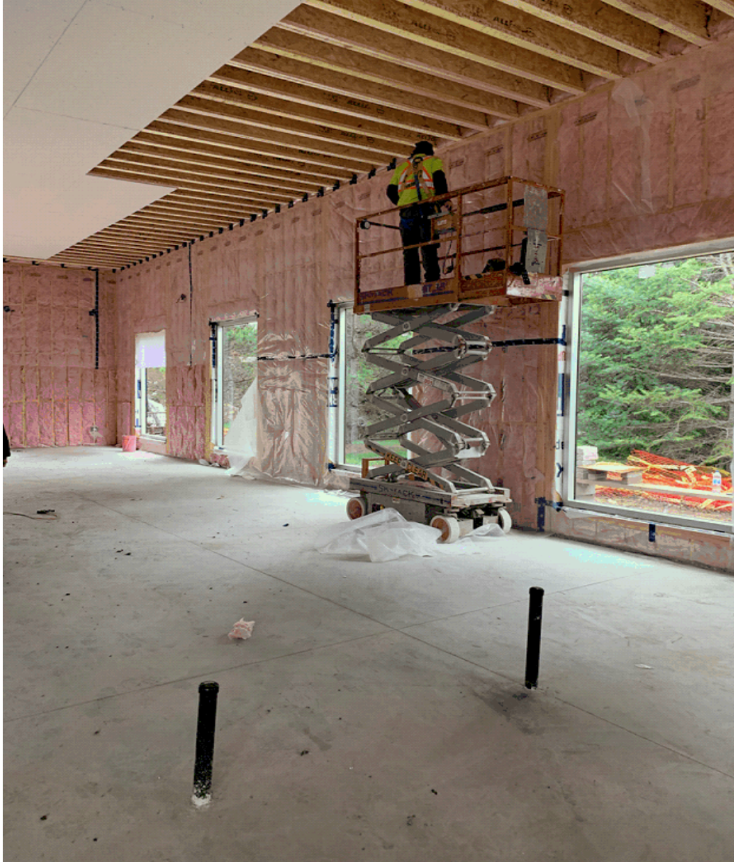
Figure 2: Daycare Addition Construction – Interior Insulation
