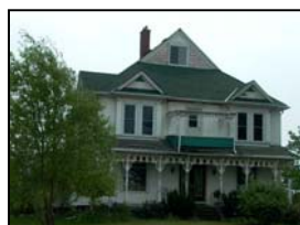
457 Queenston Road, July 2007
