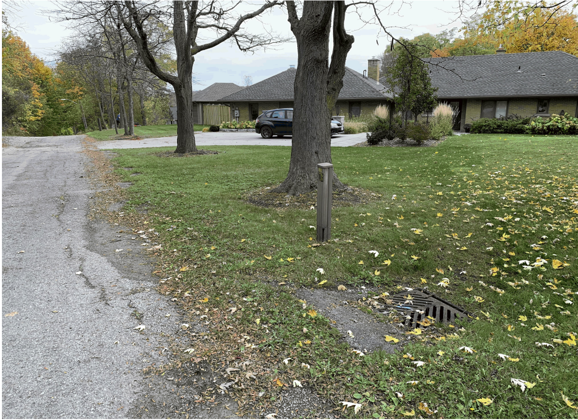
Figure 3: Catch basin on abutting property (3 Dee Road)
