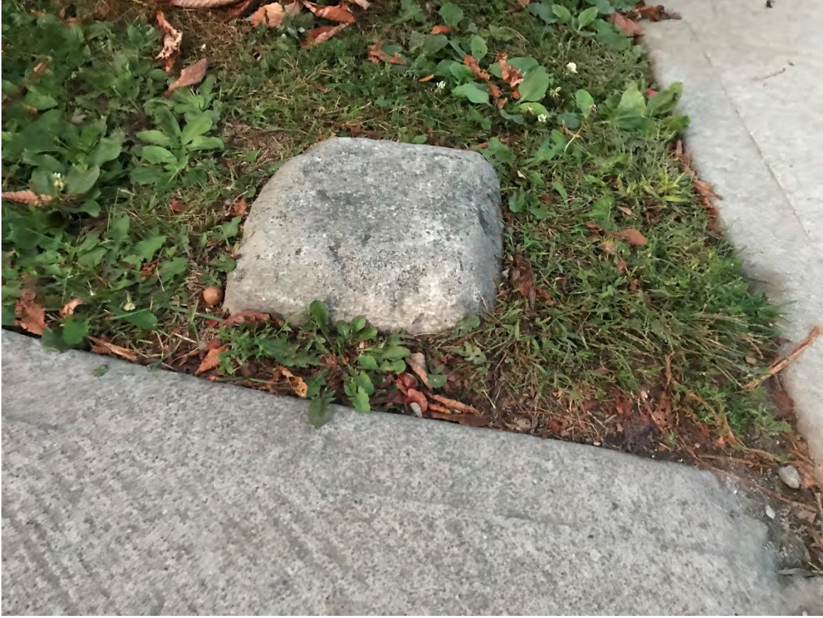
Figure 32: OBS 21 sunken down nearly flush with the ground.
