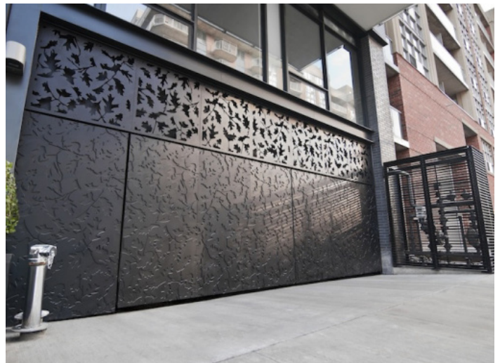
Underground parking garage access screened by decorative door
