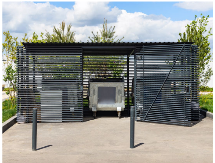
Fully enclosed garbage enclosure
