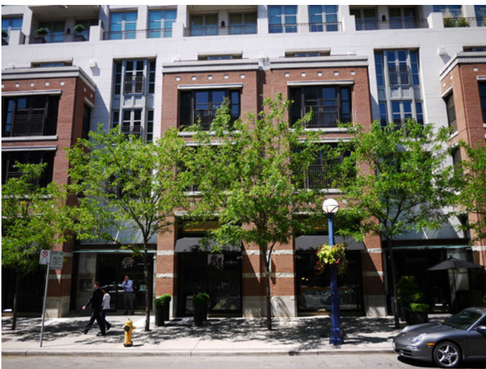
Articulation of the facade with various materials and offsets
