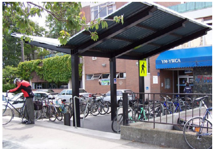
Canopy protecting bicycle parking area
