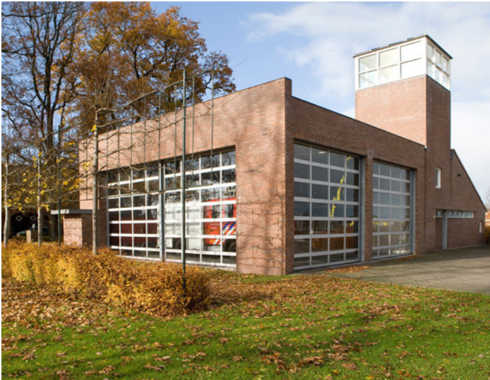
Fire station designed to integrate with and provide buffers to its surroundings
