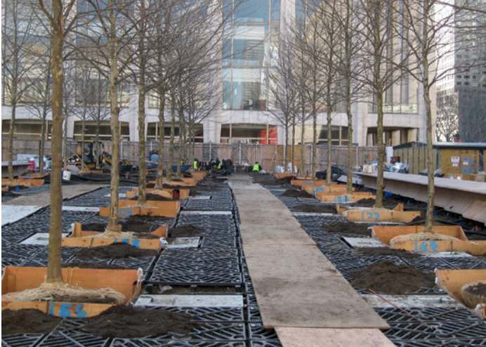
Soil cell installation at Lincoln Center New York (Source: DeepRoot on Flickr.com)
