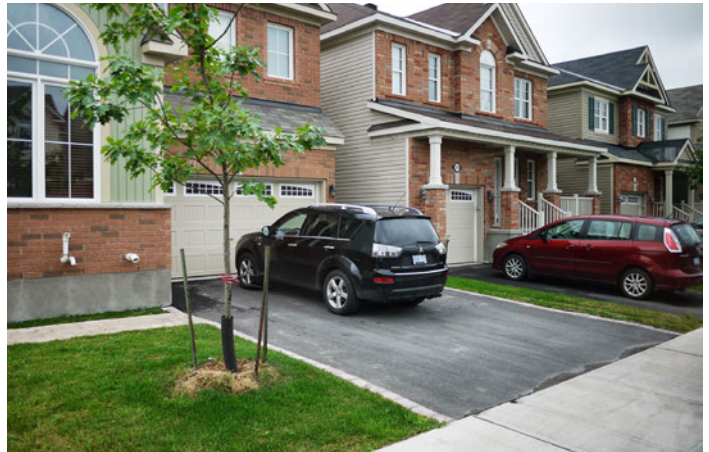
Houses with recessed front garages
