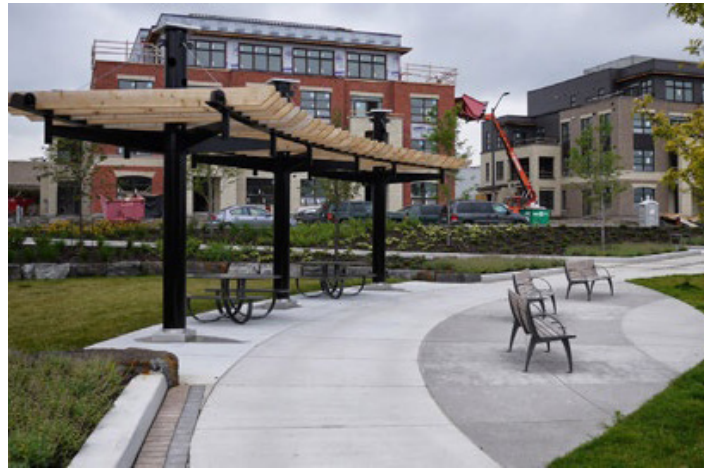
Overhead shade structure
