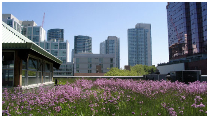
Green roof on a commercial building (Image: Sookie, CC BY 2.0, Flickr)
