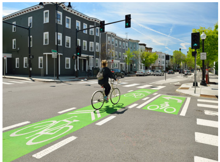
Clearly marked bike lanes through an intersection
