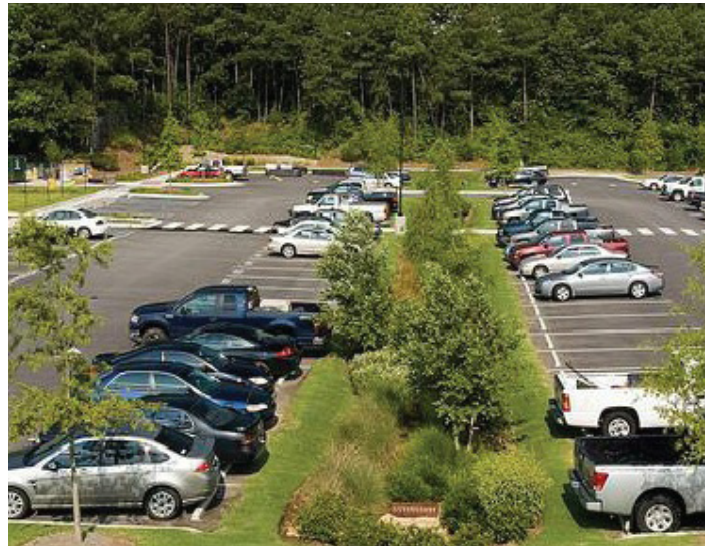
Example of a parking lot that incorporates planting strips for as a stormwater management strategy
