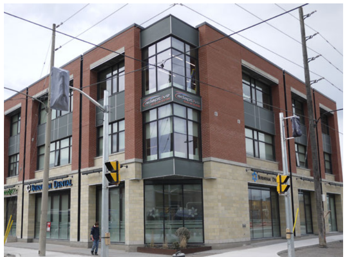
Corner articulation in a mixed use building
