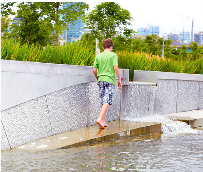
Example of an innovative stormwater management facility.
