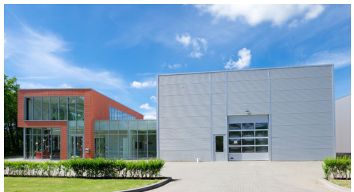
Colour, material and massing create a dynamic façade
