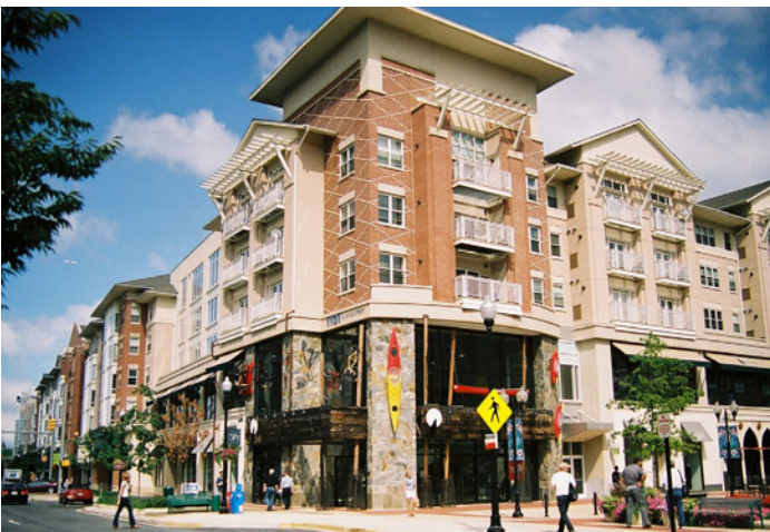
Corner building as a gateway feature
