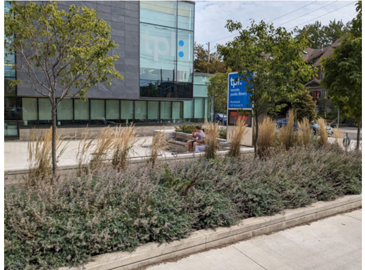
Plantings and consistent materials along the building facade
