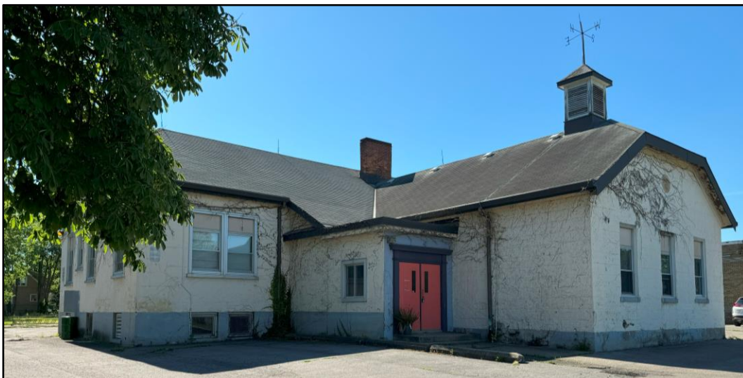
Image 6: West elevation of the 1872 one-room schoolhouse. Note that the brick chimney, and building to the rear are part of the later additions to expand the schoolhouse. A similar portal is extant on the east addition, creating entrances to separate girls and boys. These entrances replaced the central door on the south elevation.
