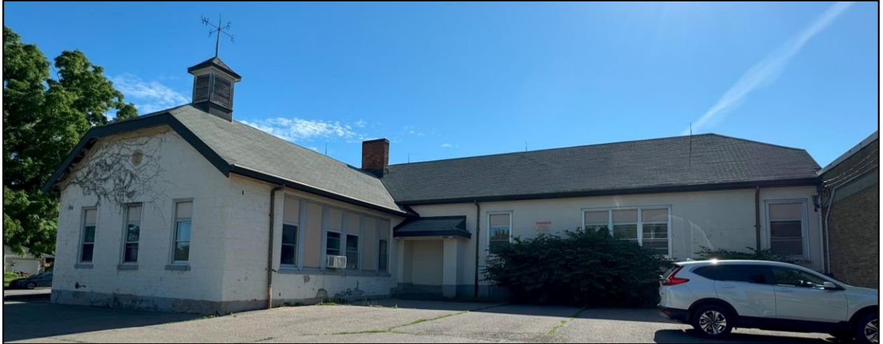
Image 9: East elevation of the 1872 one-room schoolhouse, showing the rectilinear addition that expanded across the rear of the 1872 building. The 20 th century addition has basement windows, and models the style of its opening and roof profile, albeit on a larger scale, from the 1872 design. (Image taken on: June 28, 2024)
