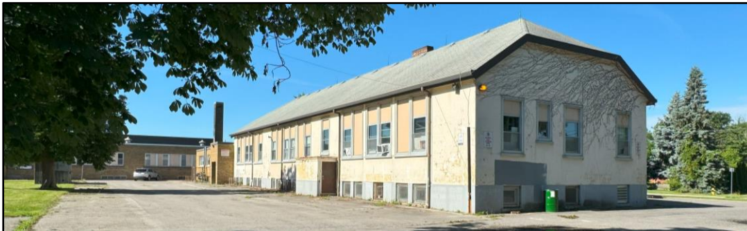
Image 8: West and north elevation of the first phases of expansion of Virgil Public School. The 20 th century addition has basement windows, and models the style of its opening and roof profile, albeit on a larger scale, from the 1872 design. In the distance, a subsequent addition clad in buff brick is visible. The land surrounding the building is paved. (Image taken on: June 28, 2024)
