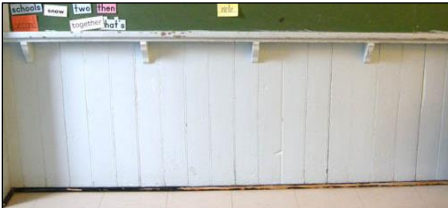
Image 16: Original wainscoting located on the interior of the 1872 one-room schoolhouse created with vertical wood planks that were later painted white. A series of evenly placed brackets creates a corbel table and ledge under the chalkboard to hold chalk, erasers, and other supplies. (Image Date: February 24, 2011)
