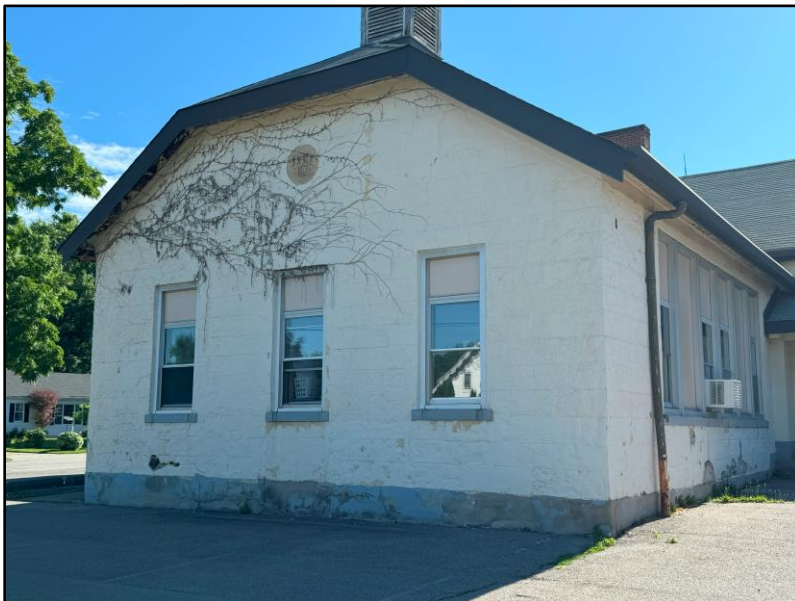
Image 2: Primary Façade (south elevation) and east elevation of the 1872 one-room schoolhouse.
