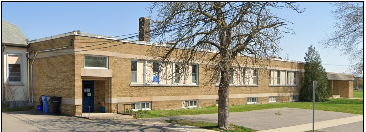
Image 12: Primary façade (south elevation) of the eastward expansion to Virgil Public School. The westernmost portion of this building projects forward, and includes a carved stone lintel over the portal that reads ‘Girls’, replacing an earlier entrance with the same functionality. Horizontal stone lintels and stringcourses emphasize the rectilinearity of the buff brick clad building. This image also illustrates the narrow depth of the setback from the sidewalk and street that was characteristic of the relationship between the original 1872 schoolhouse situated close to the public realm.
