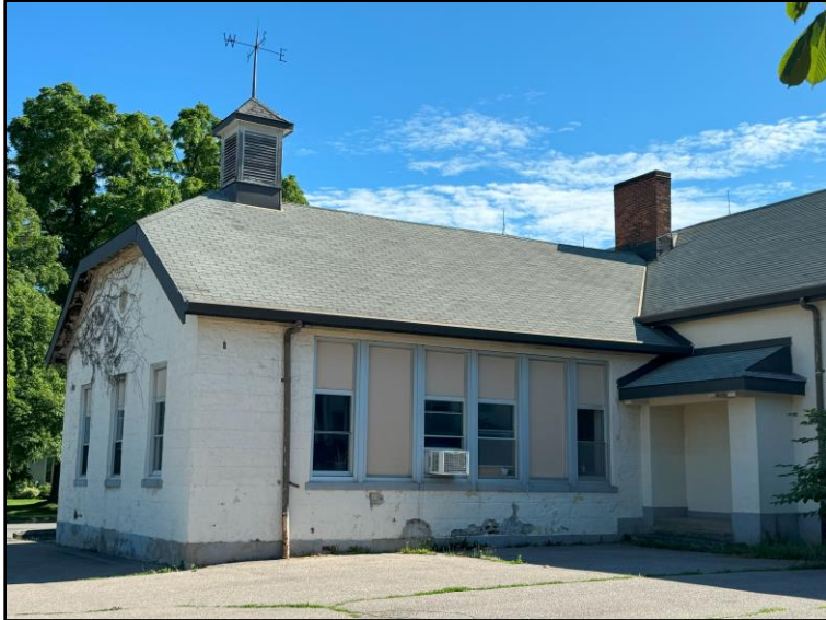
Image 5: East elevation of the 1872 one-room schoolhouse. Note that the brick chimney, and building to the rear are part of the later additions to expand the schoolhouse. A similar portal is extant on the west addition, creating entrances to separate girls and boys. These entrances replaced the central door on the south elevation.
