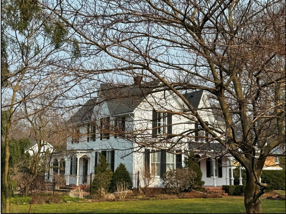
Image 3: Southwest Corner of the Residence (Image taken on: February 28, 2024)
