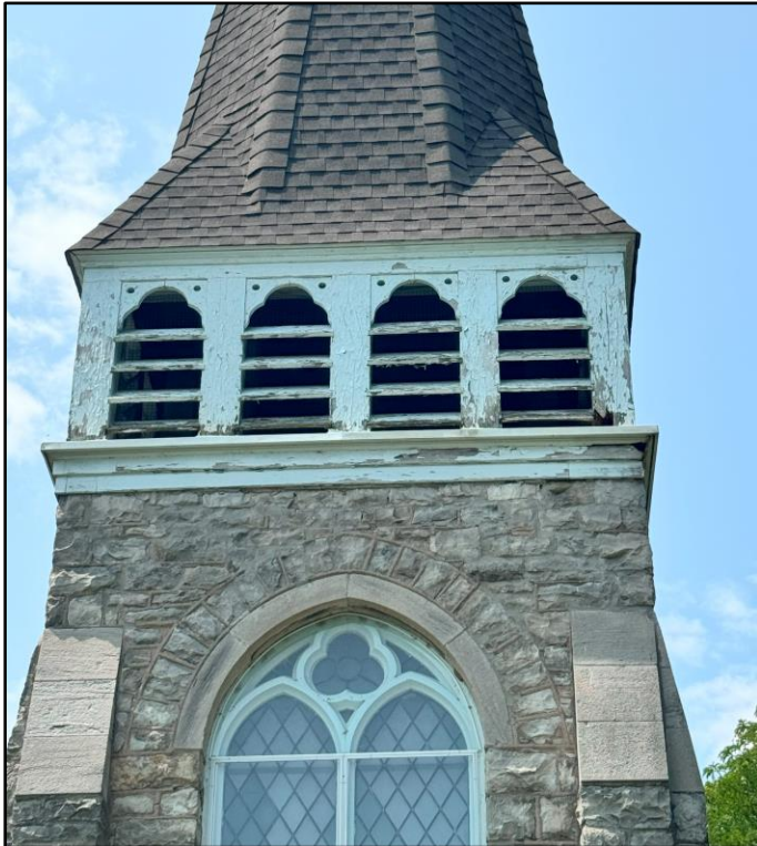
Figure 1: View of Steeple on Façade
