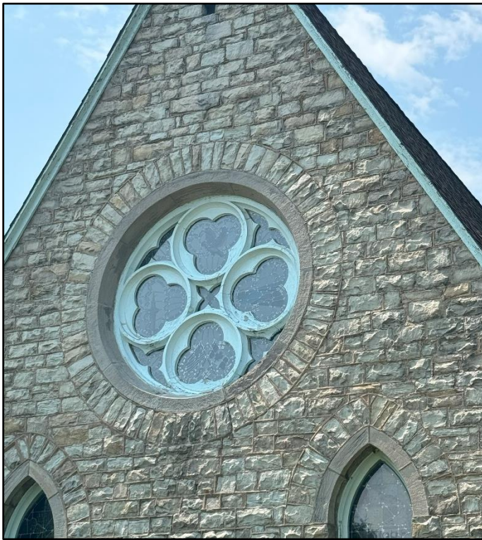
Figure 3: View of Round Window on Façade
