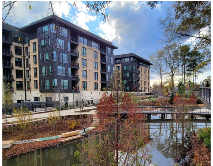
Stormwater pond at Downtown Cary Park, North Carolina Image: CC BY 2.0: Payton Chung
