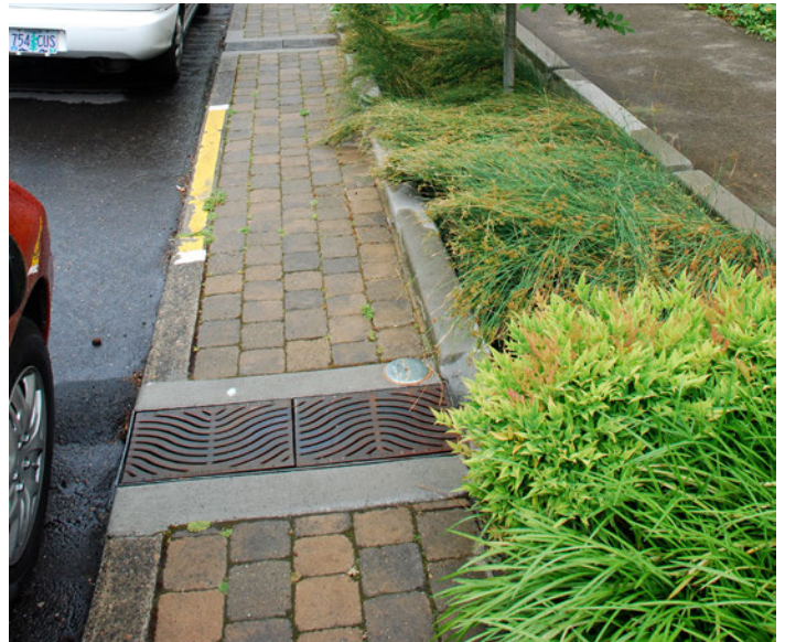
Bioretention planters for stormwater management, Portland OR
