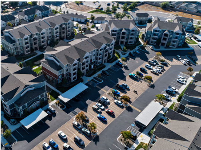
Parking for apartments with walkways and landscaping
