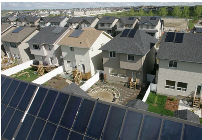
Solar panels on the roof of low-rise residential development.
