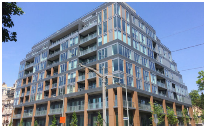
Example of a building with inset balconies to minimize shadowing on uses below
