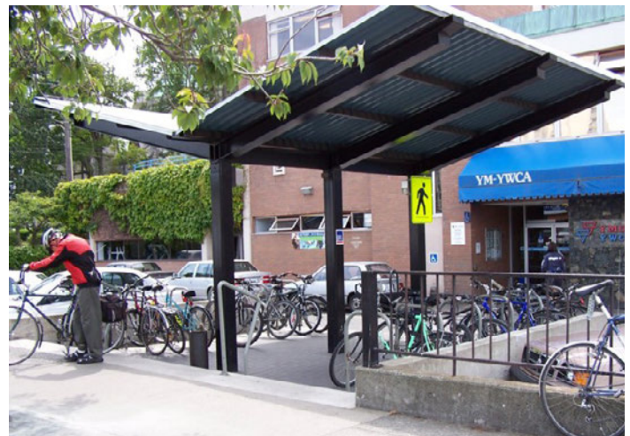
Canopy protecting bicycle parking area
