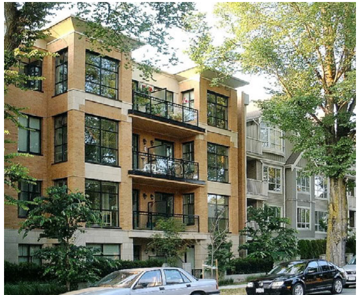
Four storey apartment building with an articulated facade
