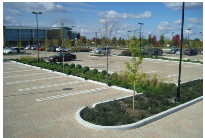
Permeable surfaces and landscaping in parking areas
