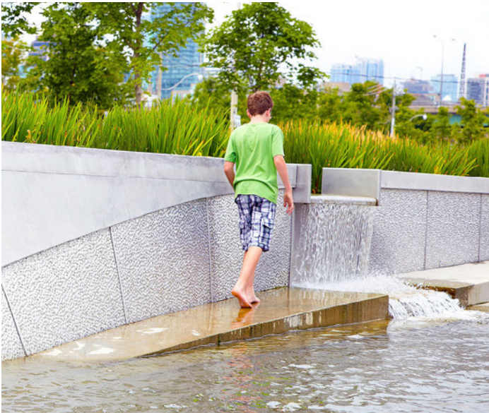
Example of an innovative stormwater management facility.
