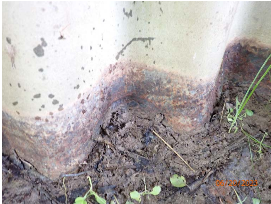
Photograph No. 4: 0277: Area of medium corrosion at the waterline (typical).
