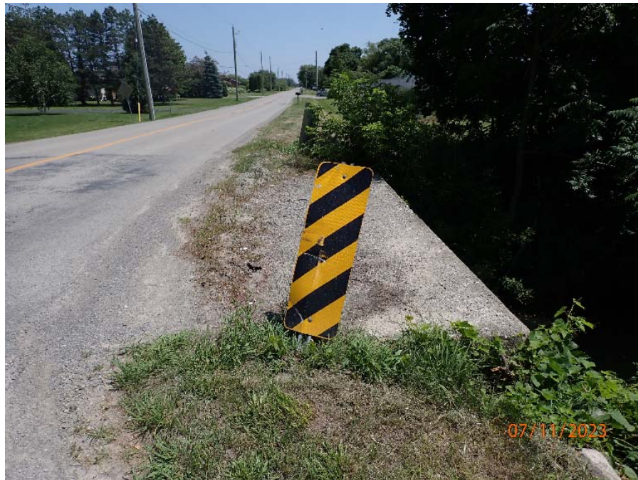
Photograph No. 4: 0582: Damaged hazard marker at southwest corner.
