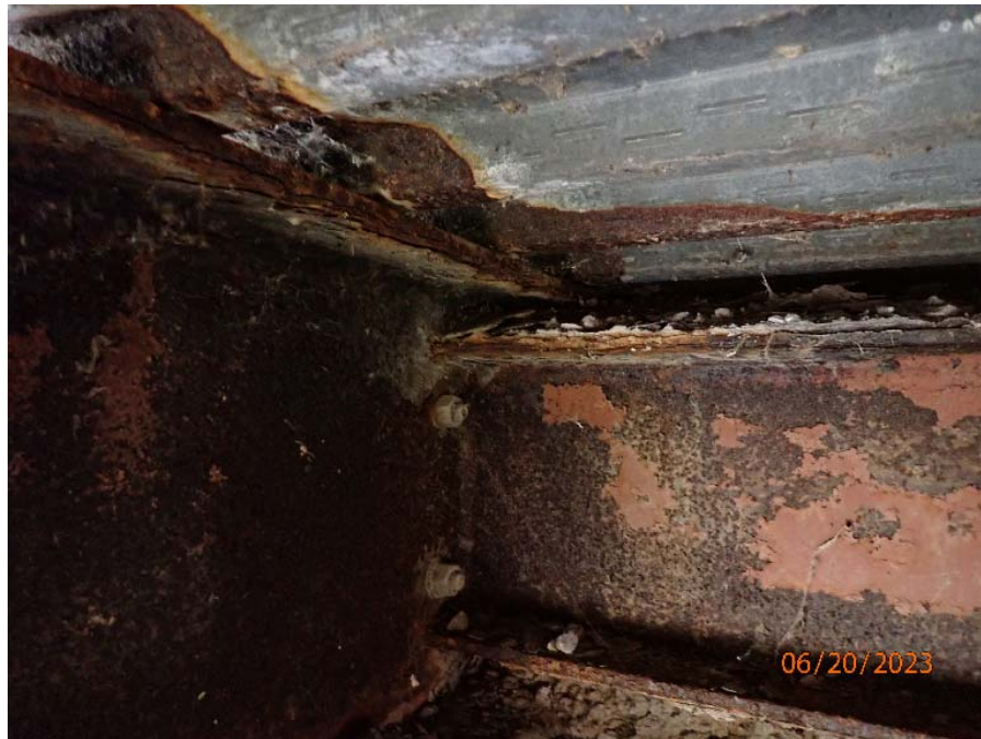
Photograph No. 4: 0778: Area of severe corrosion on west exterior girder.
