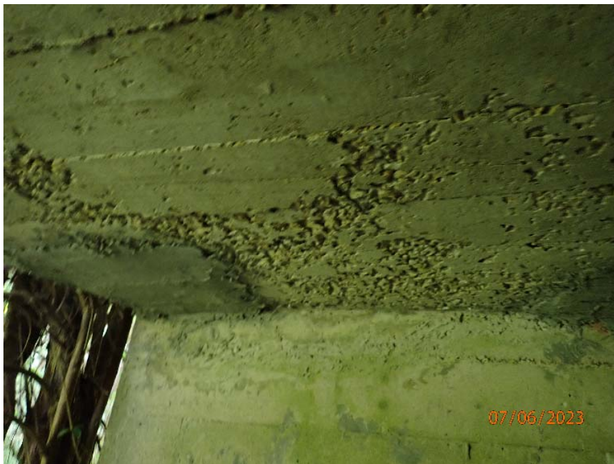
Photograph No. 4: 0387: Area of honeycombing in soffit at north end.
