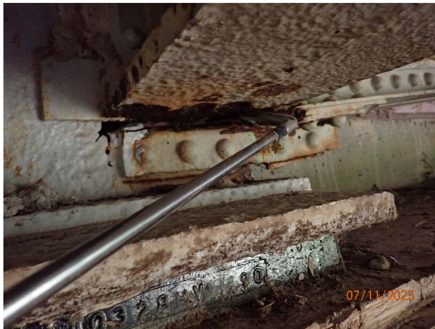
Photograph No. 4: 0885: Severe corrosion on the south exterior girder.
