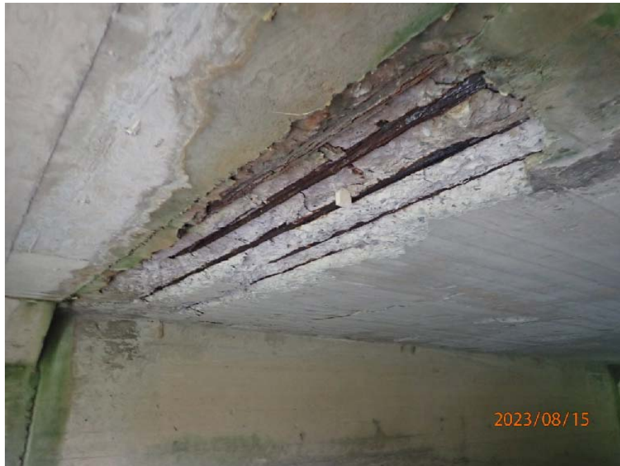
Photograph No. 4: 0618: Severe spall in the original deck soffit at the north construction joint.
