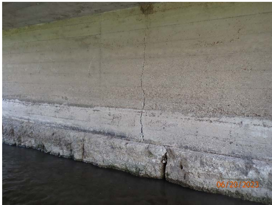
Photograph No. 4: 0441: Wide crack and exposed footings in east abutment.
