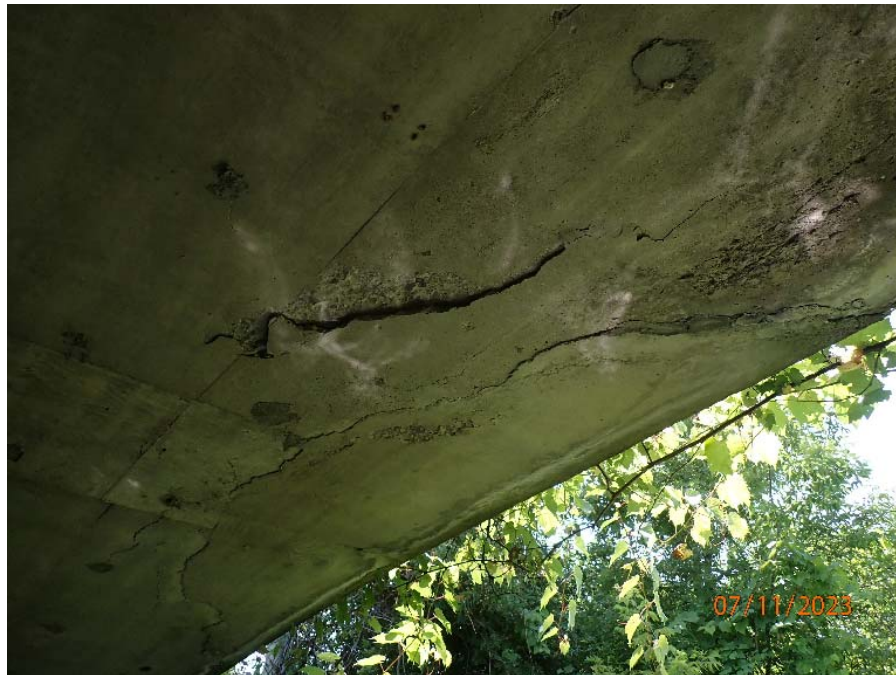
Photograph No. 4: 0437: Delamination at the south end of soffit.
