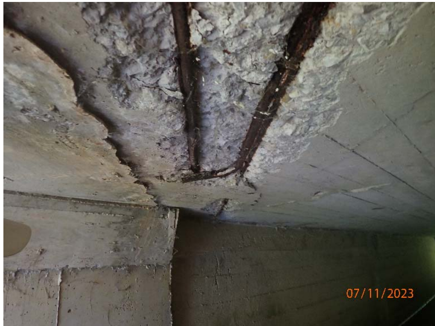
Photograph No. 4: 0162: Spall with exposed corroded reinforcing steel at the south construction joint.
