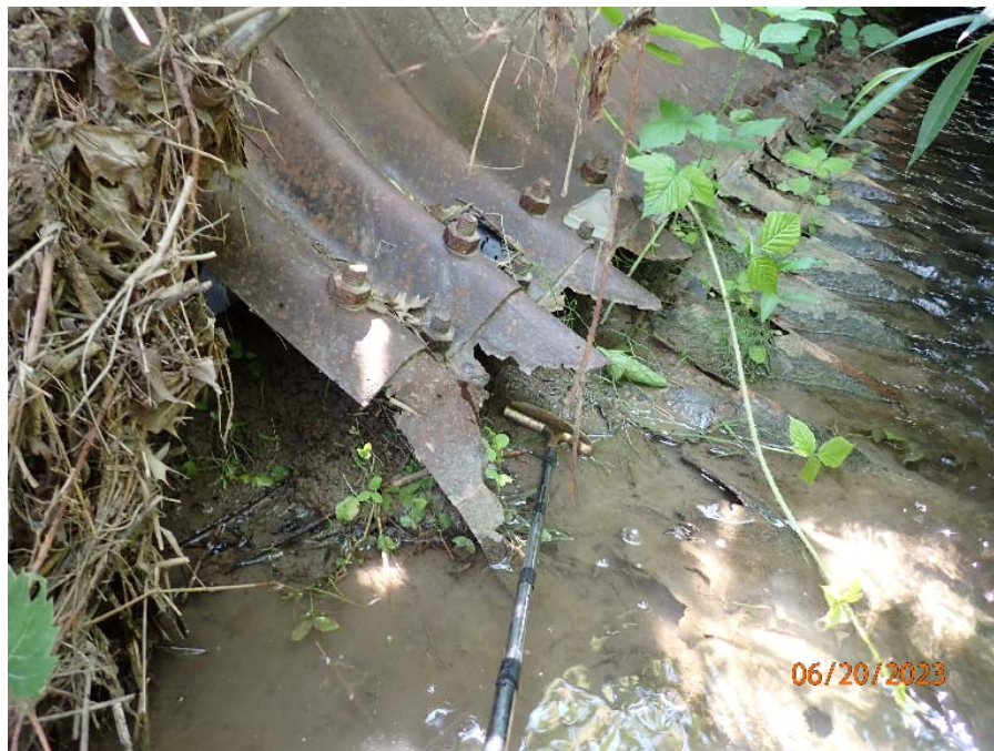
Photograph No. 4: 0545: Perforations in the north end of the west cell.
