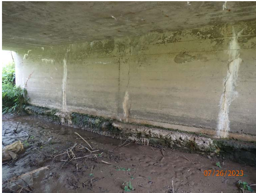
Photograph No. 4: 0416: Wide vertical cracks and efflorescent staining in abutment sidewall.
