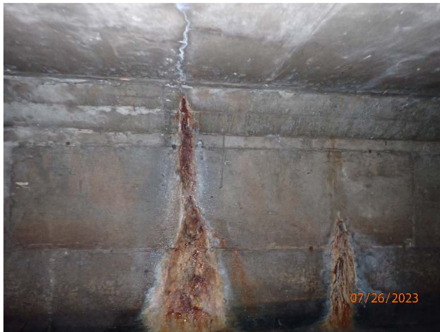
Photograph No. 4: 0090: Isolated narrow to wide cracking with efflorescent staining, rust staining, and evidence of leakage and along west abutment sidewall at centre span.
