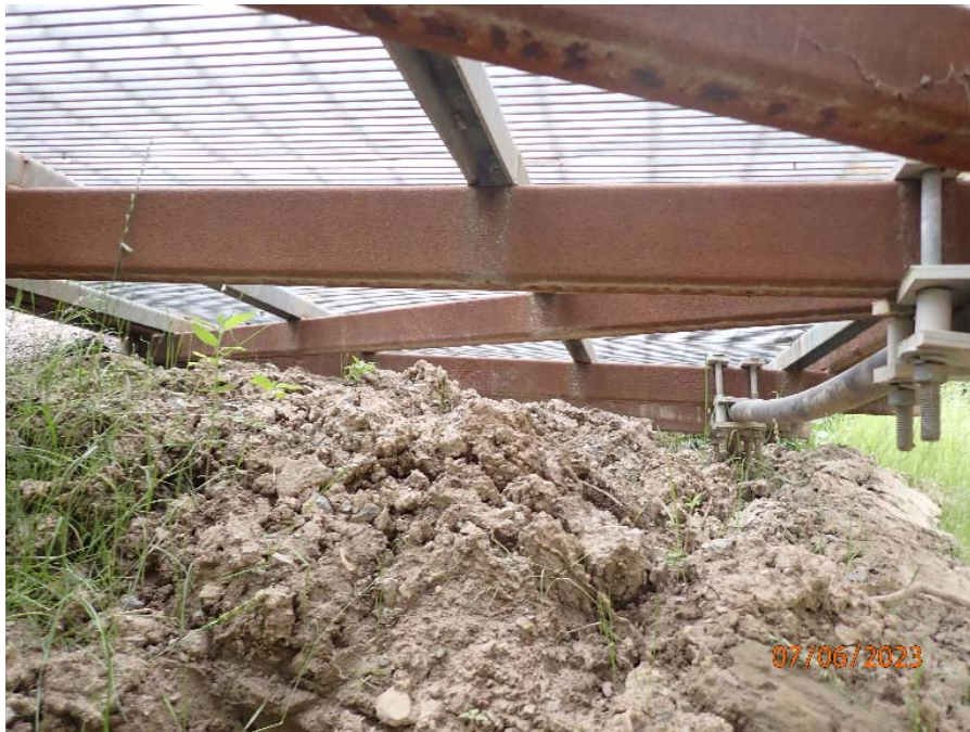
Photograph No. 4: 0809: Filled sinkhole under south end of structure, looking south.
