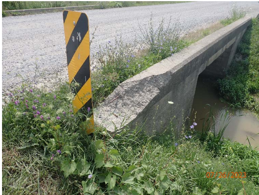
Photograph No. 4: 0626: Severe vehicular damage to northeast corner of concrete curb.
