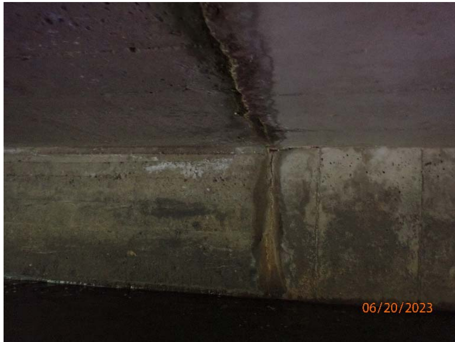
Photograph No. 4: 0103: Leakage, cracking and efflorescent staining along joint between the original structure and the east extension, looking south..
