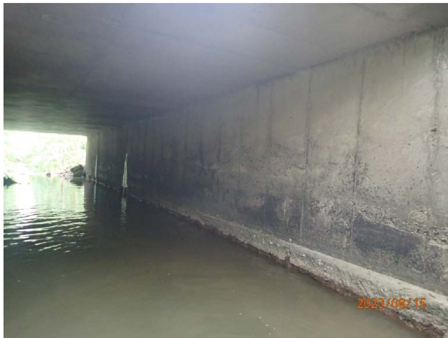
Photograph No. 4: 0407: East abutment sidewall and scour along east footing.
