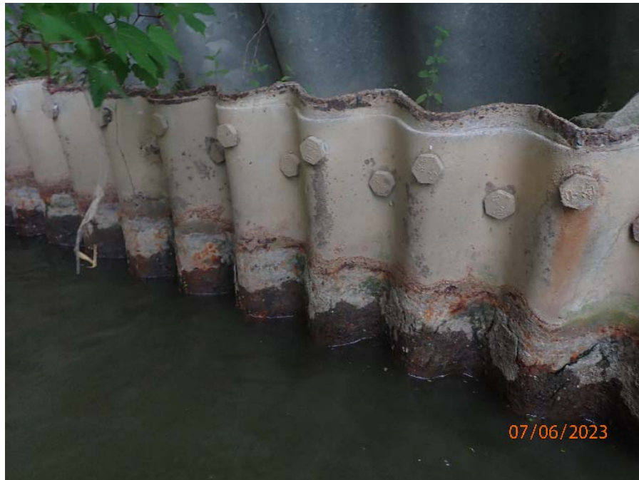
Photograph No. 4: 0649: Medium corrosion along west wall.
