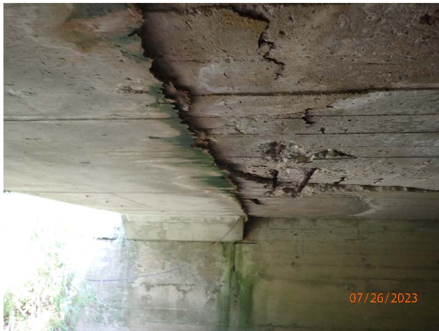
Photograph No. 4: 0723: Area of severe spalling, delamination, and exposed reinforcing steel at the north end of the original soffit.
