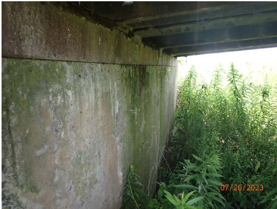
Photograph No. 4: 0698: Outward rotation in south abutment.
