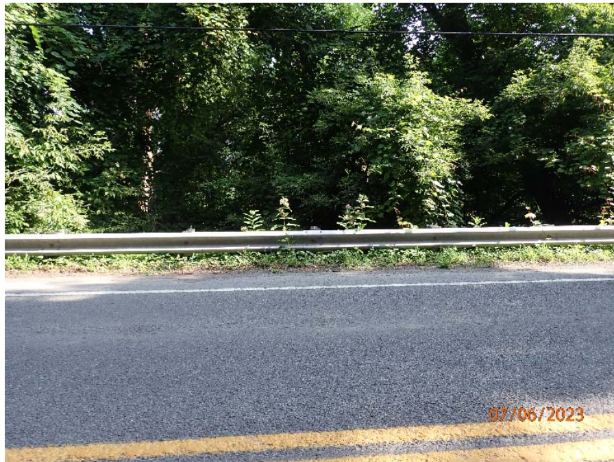
Photograph No. 4: 0089: Low guiderail at north side of roadway.
