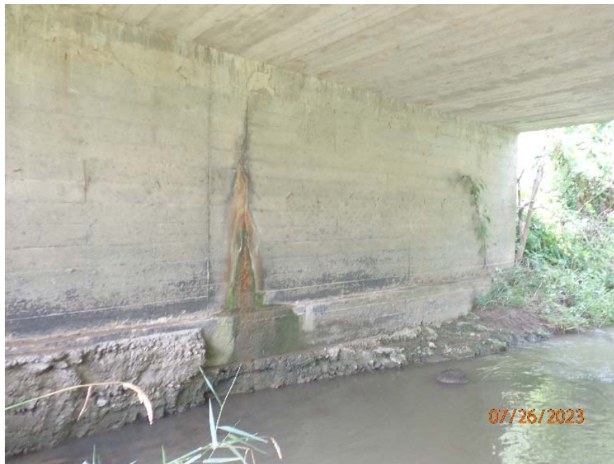
Photograph No. 4: 0550: Severe scour, wide crack with efflorescent staining and active leakage on west abutment.
