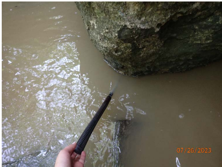
Photograph No. 4: 0290: Undermining at northeast corner.
