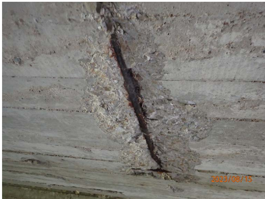
Photograph No. 4: 0449: Spall with exposed corroded reinforcing steel at the centre-span of the soffit.
