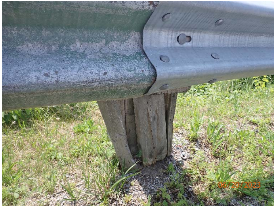
Photograph No. 4: 0588: Split timber post (typical).
