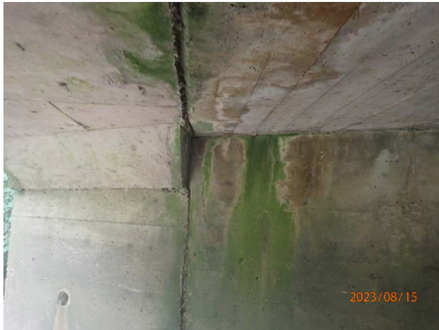
Photograph No. 4: 0551: Evidence of leakage and staining at the construction joint (typical).
