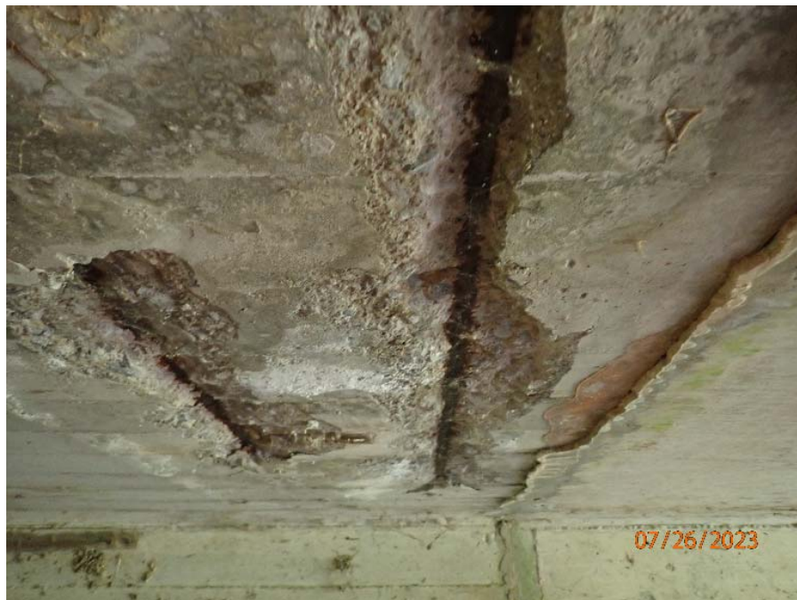
Photograph No. 4: 0487: Severe spall at south end of original portion of the soffit.
