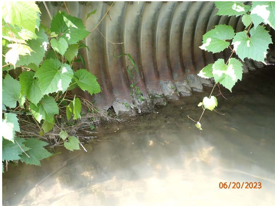
Photograph No. 4: 0619: Severe corrosion and perforations at southeast corner in the west cell.
