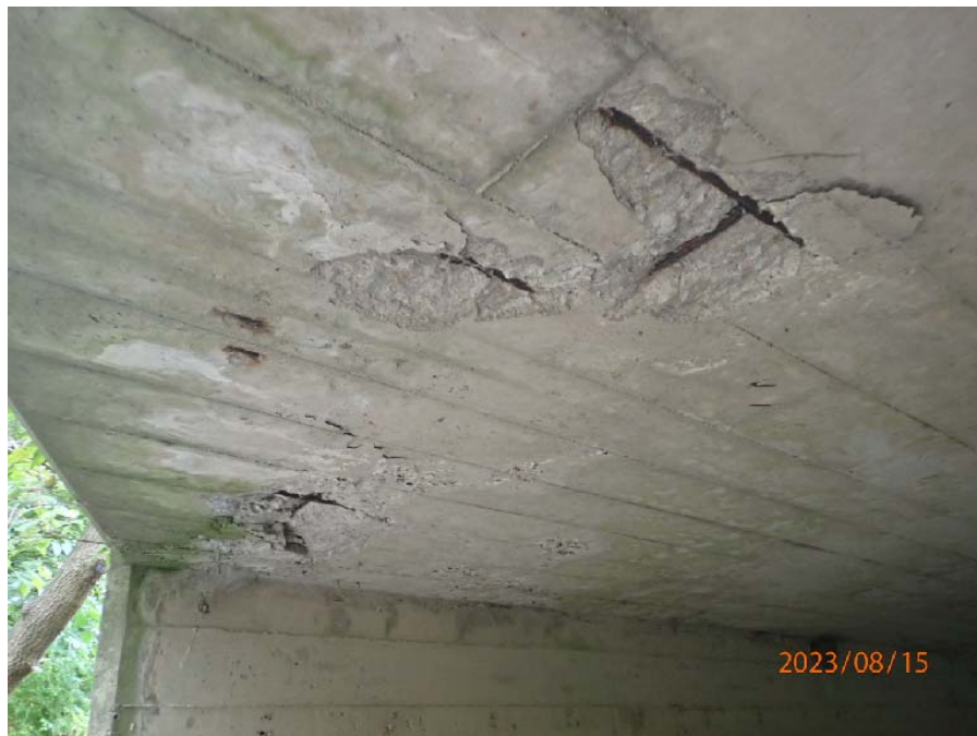
Photograph No. 4: 0678: Area of delamination, exposed corroded reinforcing steel and efflorescent staining at the south end.
