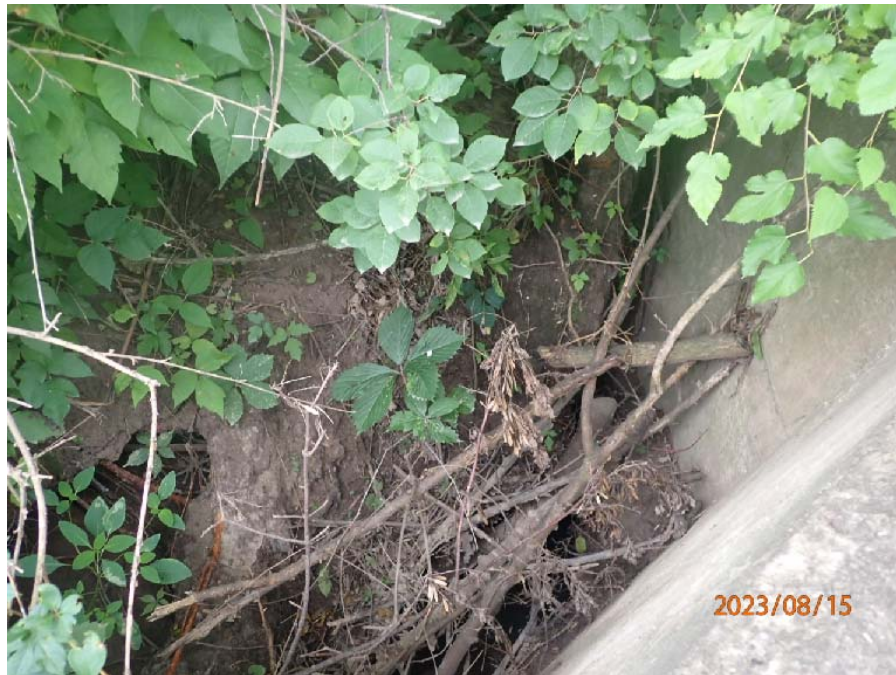
Photograph No. 4: 0286: Severe erosion behind southeast wingwall.
