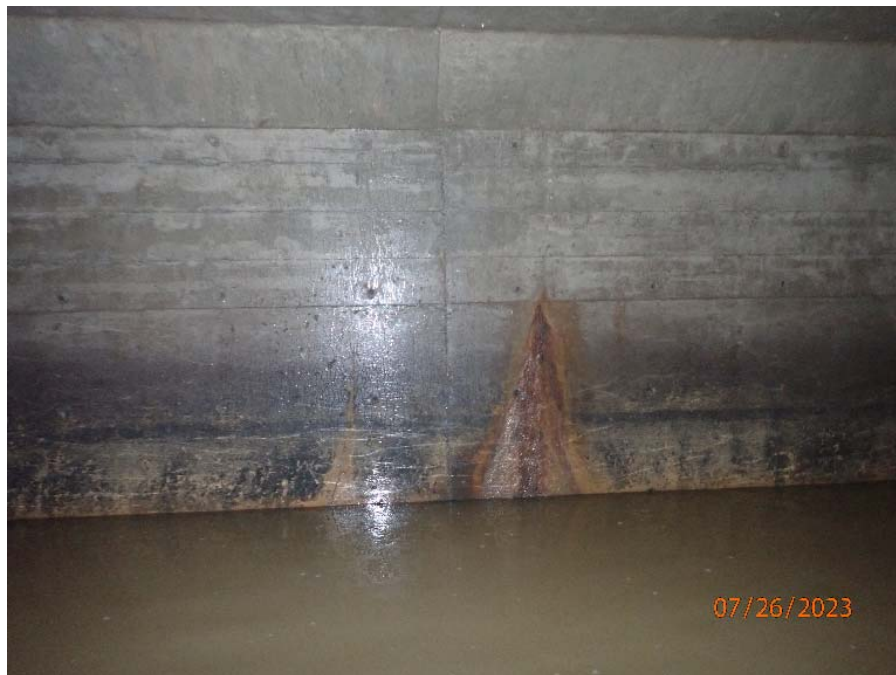
Photograph No. 4: 0356: Area of cracking, efflorescent staining, and active leakage in abutment sidewall.
