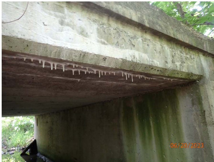
Photograph No. 4: 0898: Efflorescent staining, active leakage and stalactites at north fascia/curb.
