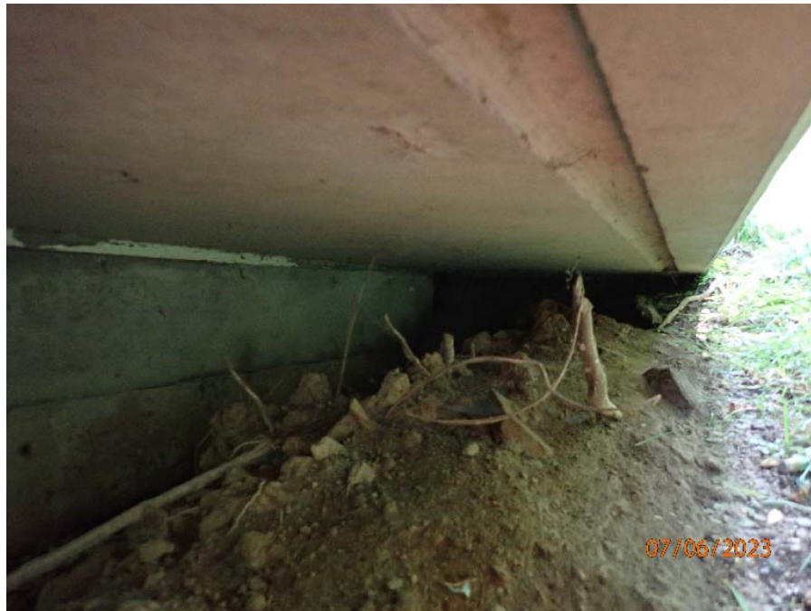
Photograph No. 4: 0232: Medium erosion and possible underpinning at southeast cantilever.
