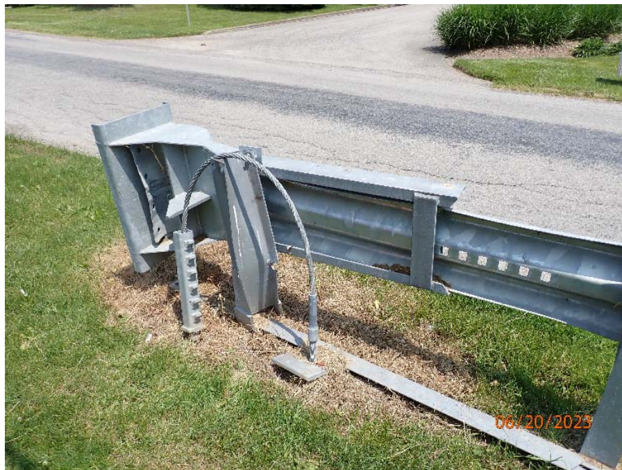
Photograph No. 4: 0746: Damaged end treatment at northwest corner.
