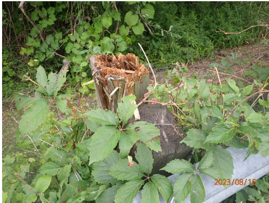
Photograph No. 4: 0211: Rotted and rotated timber posts (typical).
