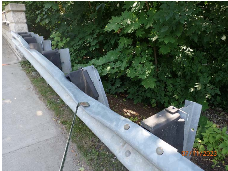
Photograph No. 4: 0472: Damage to the steel beam guiderail at southwest corner.
