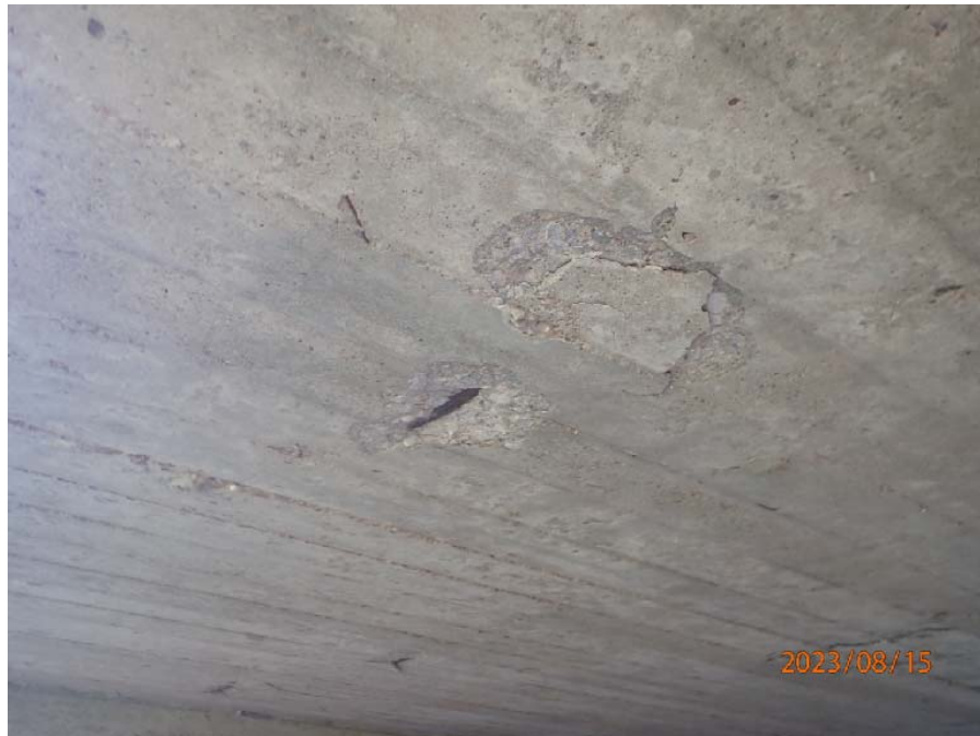
Photograph No. 4: 0512: Spalling and delaminations with exposed corroded reinforcing steel in soffit.
