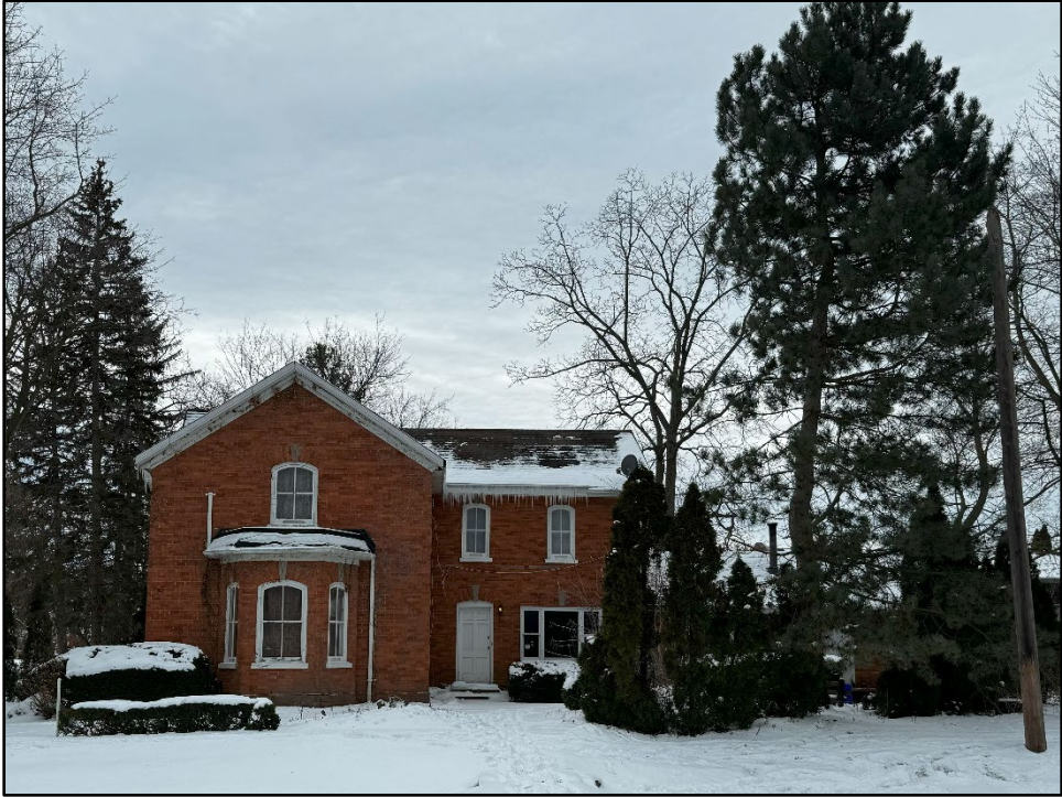
Image 3: North Elevation of Best house (Image taken on: January 22, 2024)
