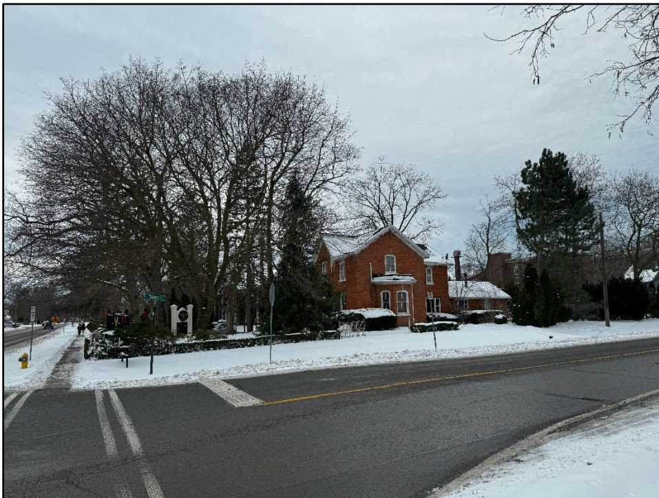
Image 10: View of the Subject Property at the Intersection of King Street and Mary Street (Image taken on: January 22, 2024)
