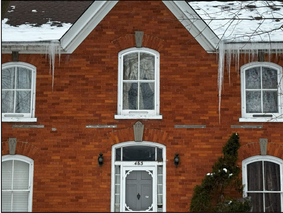
Image 5: Brick Voussoirs and Keystone Details on Façade (Image taken on: January 22, 2024)
