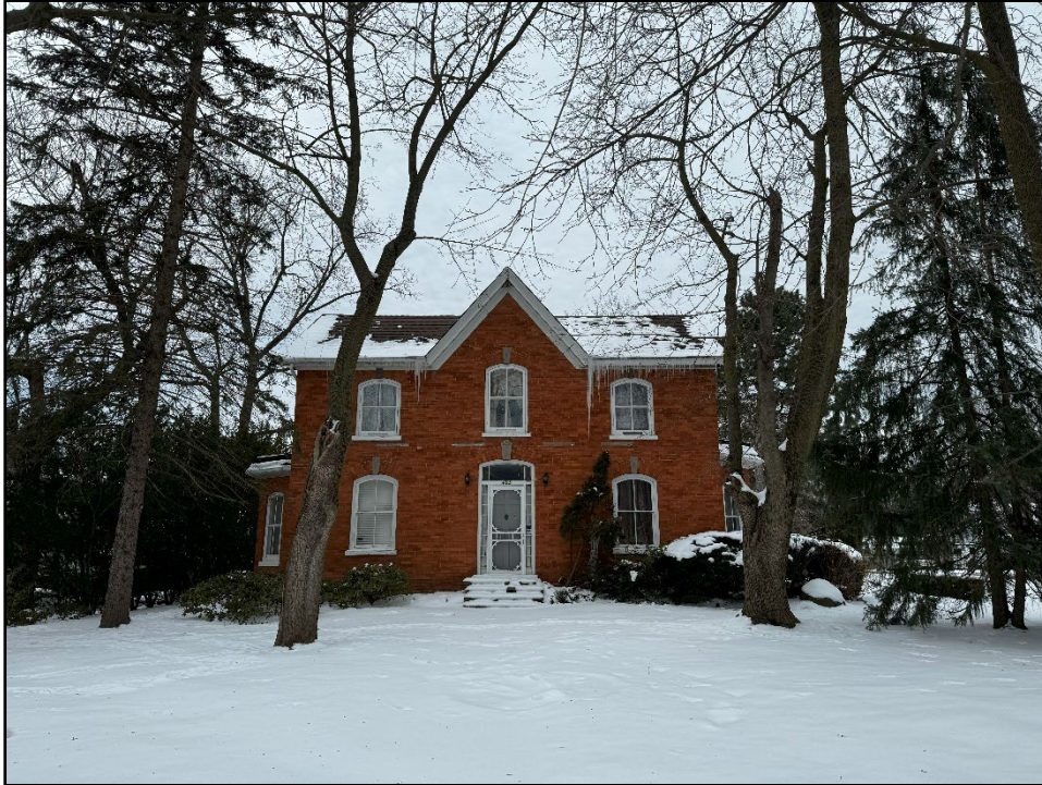
Image 1: Facade (East Elevation) of Best House (Image taken on: January 22, 2024)
