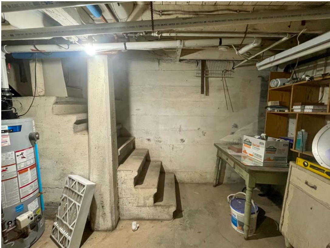
REAR ADDITION BASEMENT – poured-in-place concrete foundation below the coatroom
