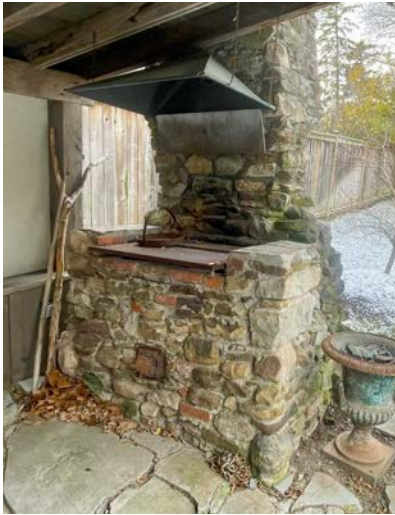
OPEN GARDEN STRUCTURE – built-in barbeque built with salvaged stone & brick – wood frame built with salvaged beams and dimensioned lumber
