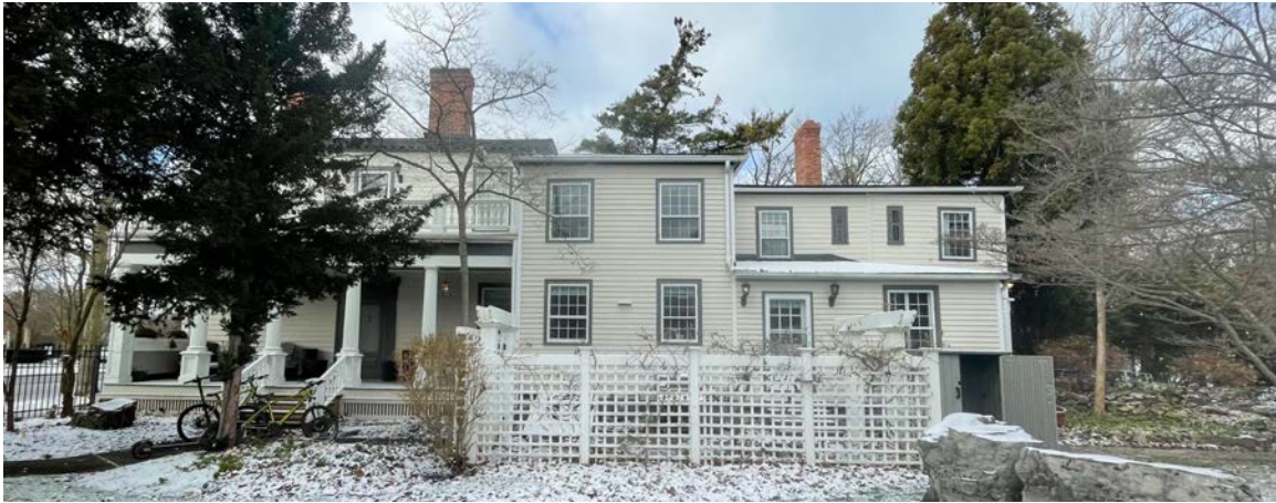
SIDE ELEVATION – the main entrance to the house is through the porch on the side elevation
