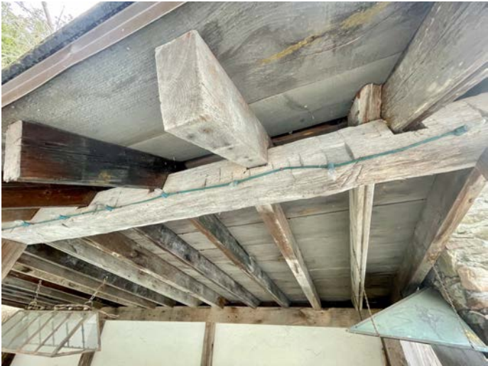
OPEN GARDEN STRUCTURE – built-in barbeque built with salvaged stone & brick – wood frame built with salvaged beams and dimensioned lumber
