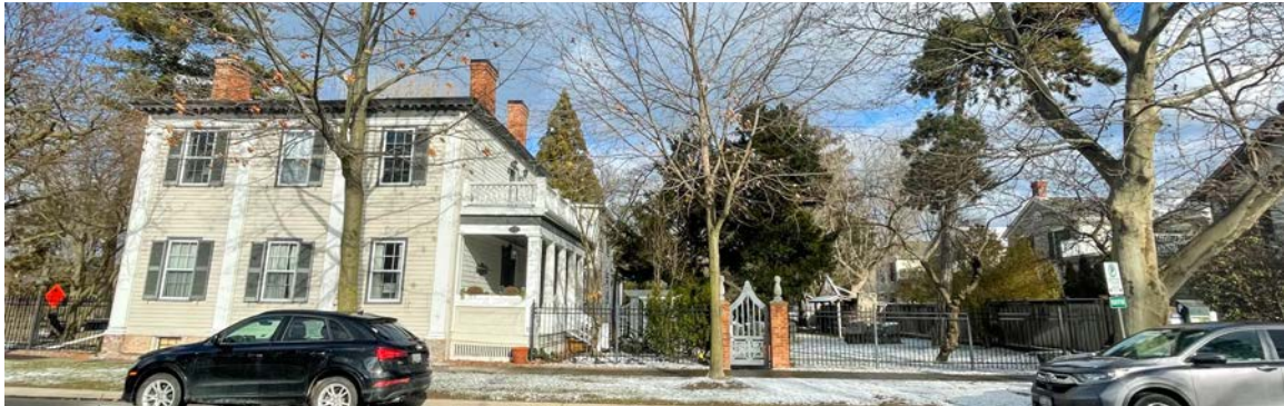
QUEEN STREET ELEVATION – the main entrance to the house is oriented towards the south side yard
