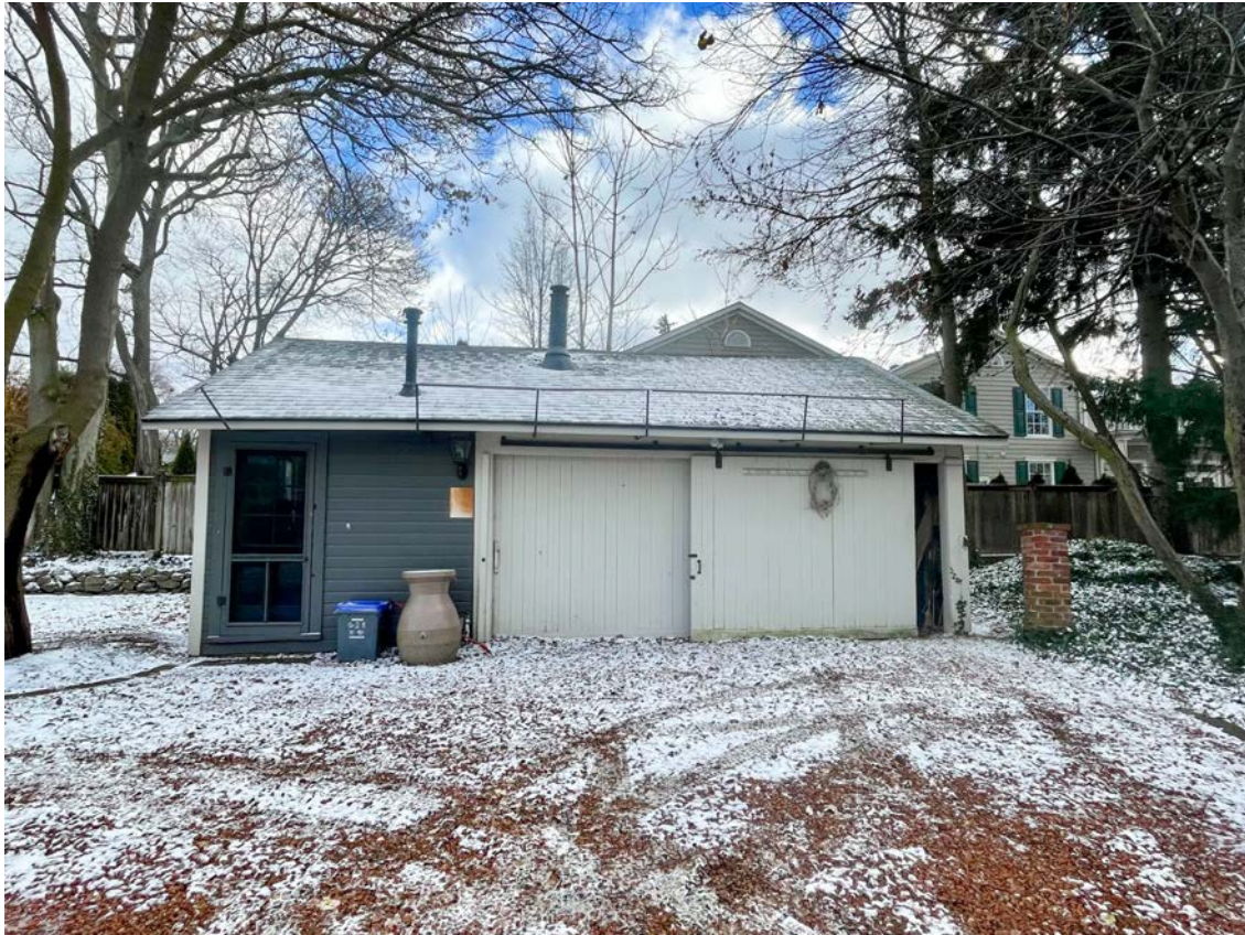
DETACHED GARAGE – wood frame building with wood siding
