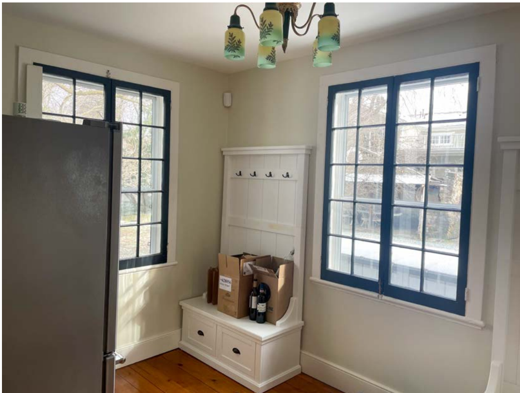
REAR ADDITION INTERIOR: interior of the coatroom – double-casement style wood windows
