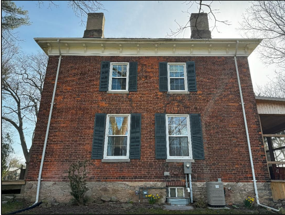
Image 7: West Elevation of Roselawn (Image taken on: April 9, 2024)
