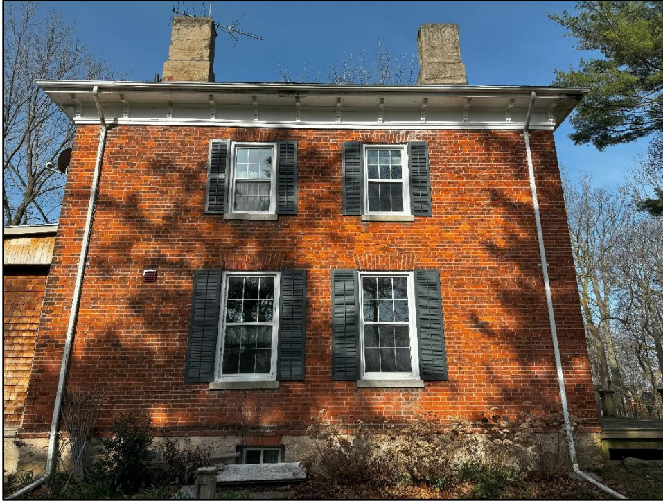
Image 3: East Elevation of Roselawn (Image taken on: April 9, 2024)
