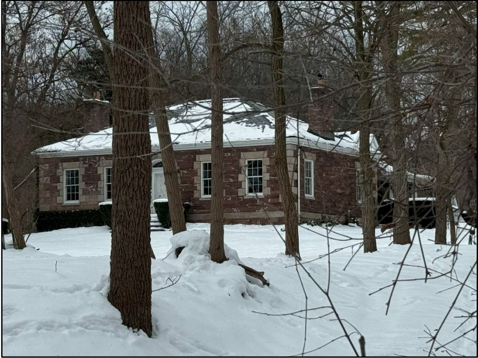
Image 2: Northwest Corner of Warner House (Image taken on: January 22, 2024)
