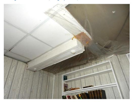
Figure 35: 200 John Street, Garage Apartment, Beaver Board Walls, False Ceiling and Ceiling Damage
