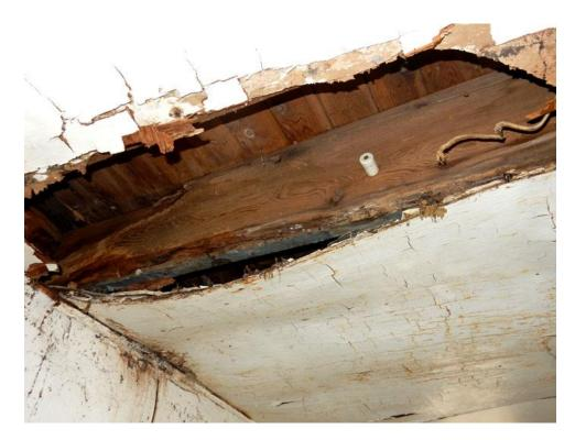
Figure 58: 200 John Street, Pool House, Ceiling Damage
