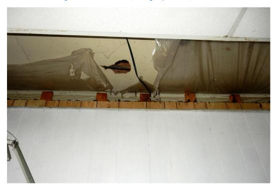
Figure 33: 200 John Street, Garage Apartment, Bedroom Ceiling Damage and Beaver Board Walls
