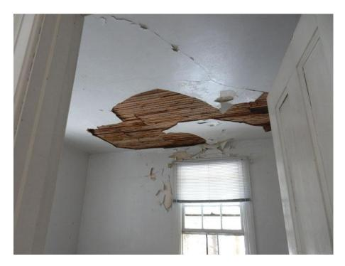
Figure 30: 200 John Street, Garage, Ceiling Damage
