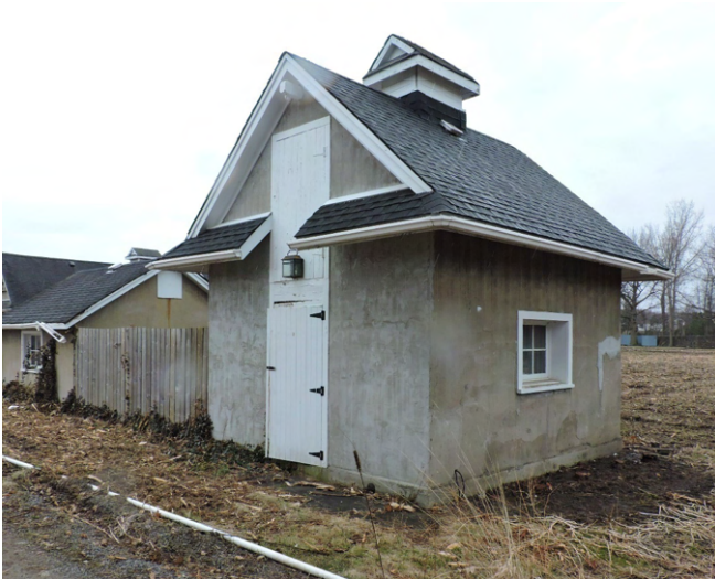
Figure 24: Northern shed (LHC, 2019)
