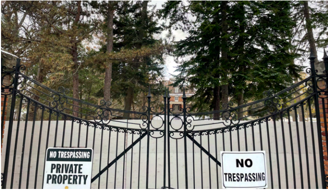
Figure 6: View of 176 John Street East
