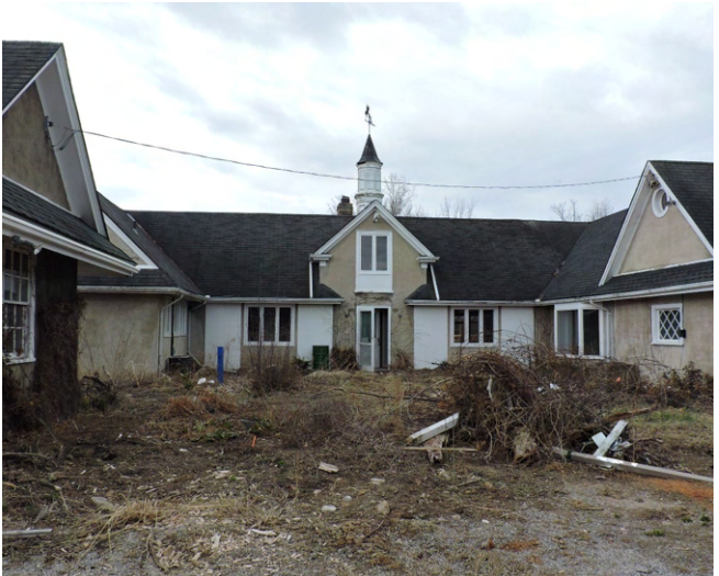
Figure 25: Former stables (Main House) (LHC, 2019)
