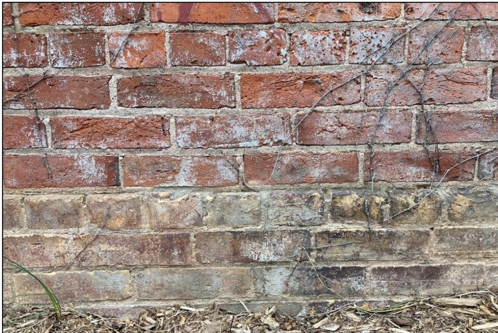
Photograph 14: Detail of buff brick foundation and Common bond brick construction (WSP, 2023)
