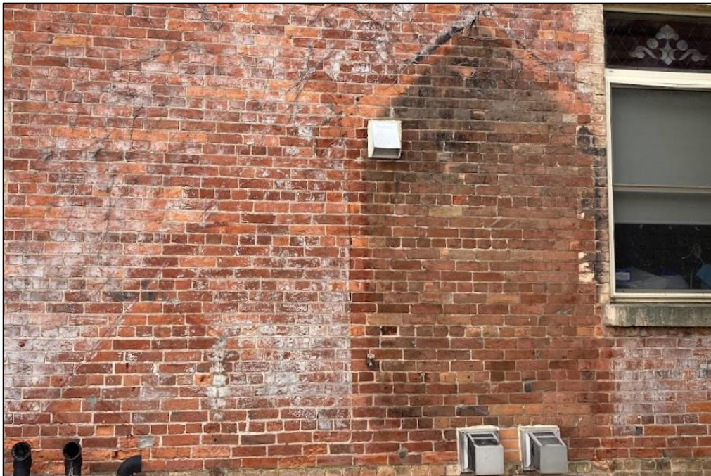
Photograph 22: Ghosting on brick from former cold room on the west façade (WSP, 2023)
