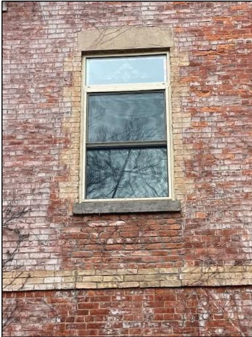
Photograph 12: Detail of second storey door converted to a window (WSP, 2023)
