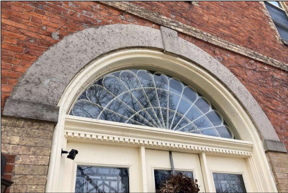
Photograph 5: Detail of fanlight with tracery and cut stone lintel with projecting keystone (WSP, 2023)
