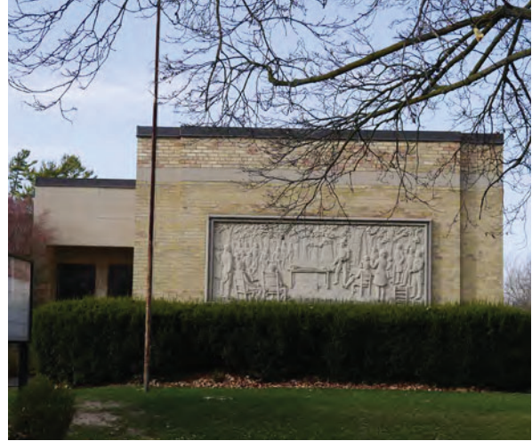
11. View of the northern bas-relief stone panel at the primary (east) elevation of the original 1948 structure (Source: ERA Architects).
