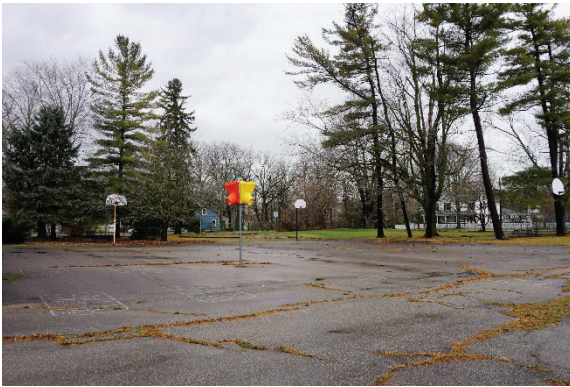
Photo 4.3: Pavement area, looking southwest
