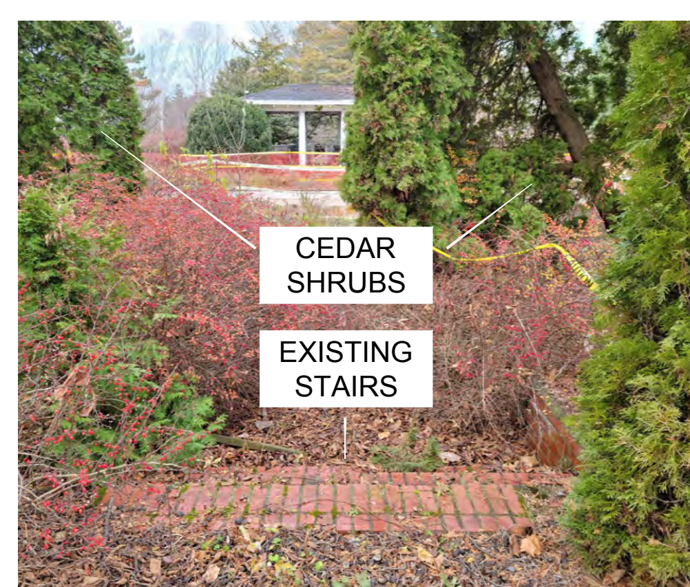
2A L1 EXISTING STAIRS AND CEDAR SHRUBS SITE VISIT PHOTO
