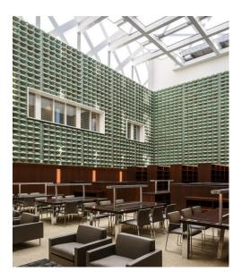
Plate 3.3: Salvaged copper roofing material used as acoustic wall treatment, Ottawa, Ontario Display of Salvaged Materials
