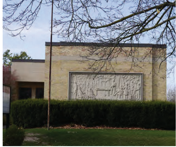
11. View of the northern bas-relief stone panel at the primary (east) elevation of the original 1948 structure (Source: ERA Architects).
