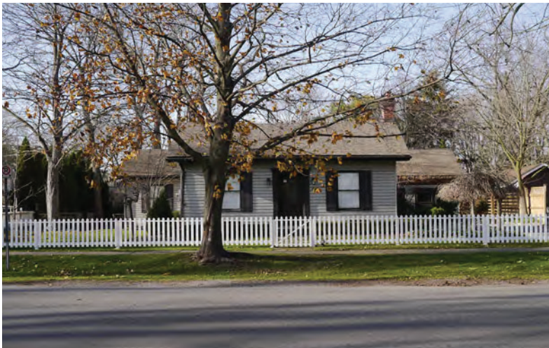
22. Adjacent heritage resource at 327 Regent Street (Source: ERA Architects).
