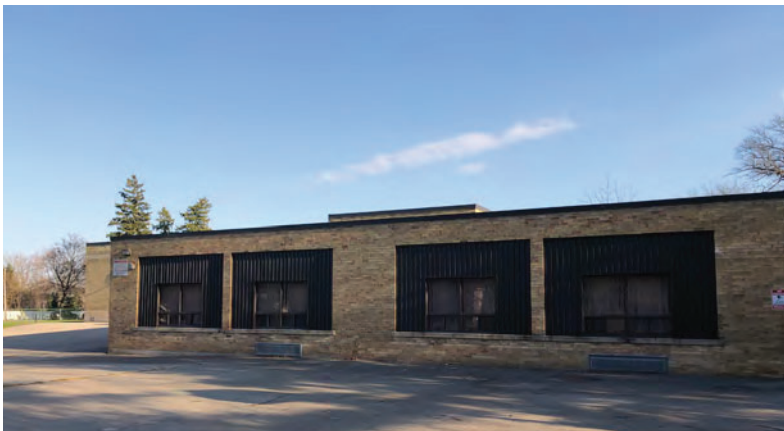
16. View of the rear (west) elevation of the 1956 addition (Source: ERA Architects).
