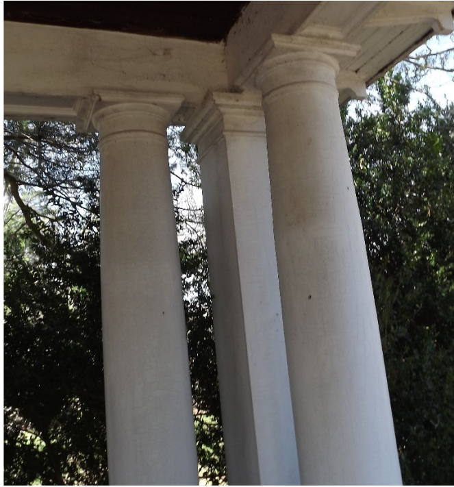
Corner columns in good condition
