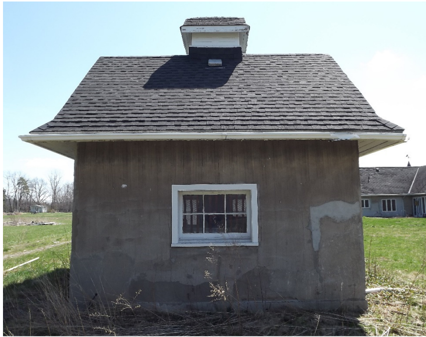
Shed D West elevation
