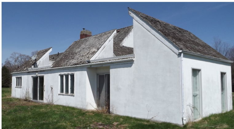
Guest House Southeast Aspect
