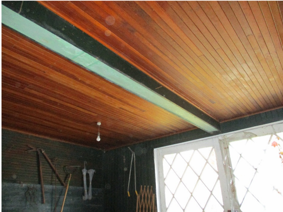
Ceiling detail in workshop
