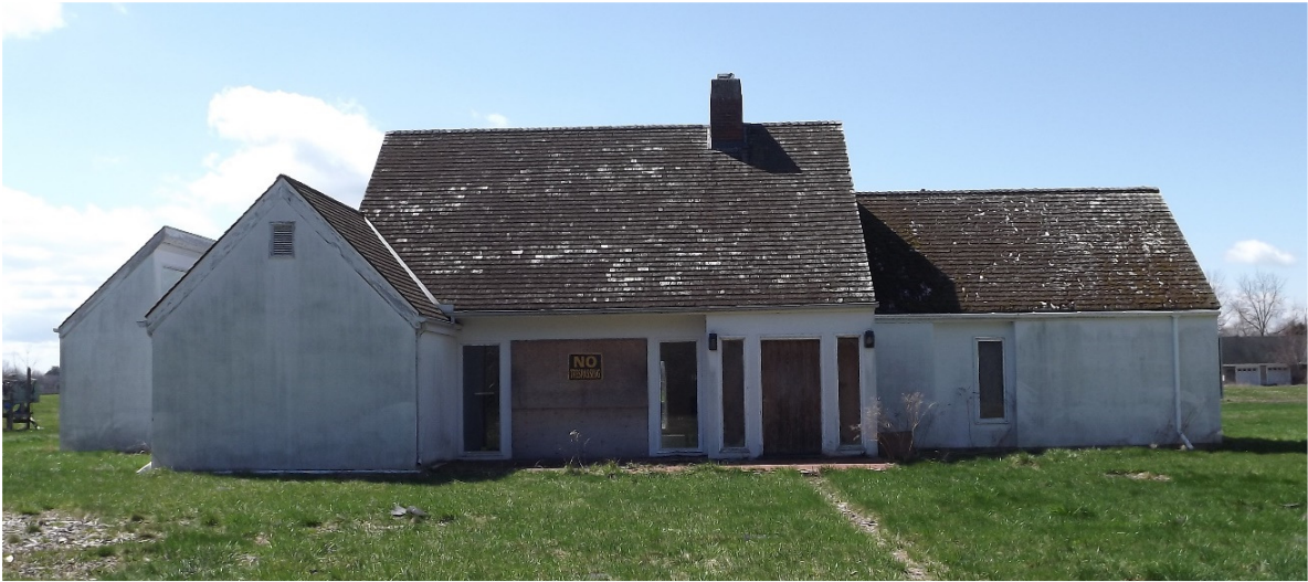
The Guest House North Elevation, April 2022
