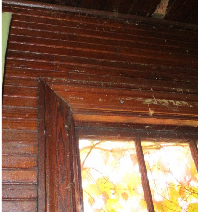
Detail showing fir panelling, window casing, and sash in garage
