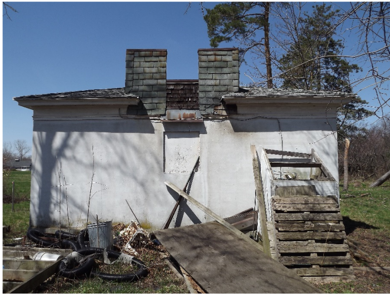
Rear wall of Bath House showing roof platform
