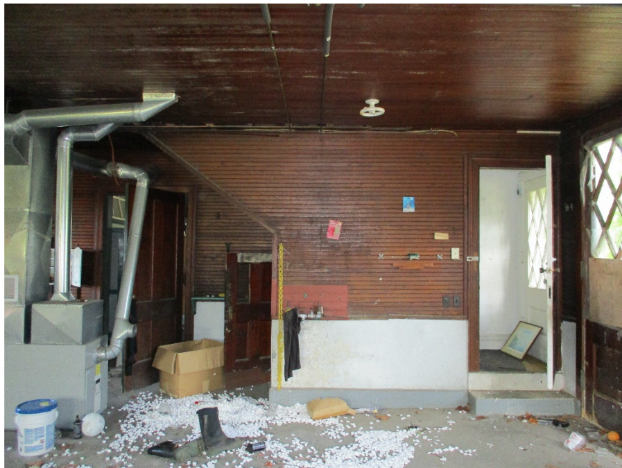
Interior of garage; note new furnace, door to apartment
