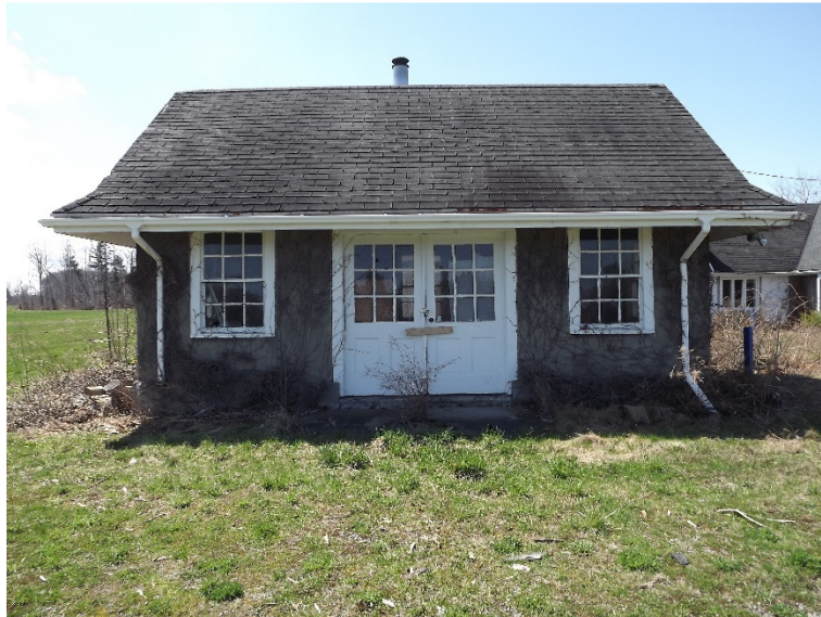
North Elevation of Building B - Workshop
