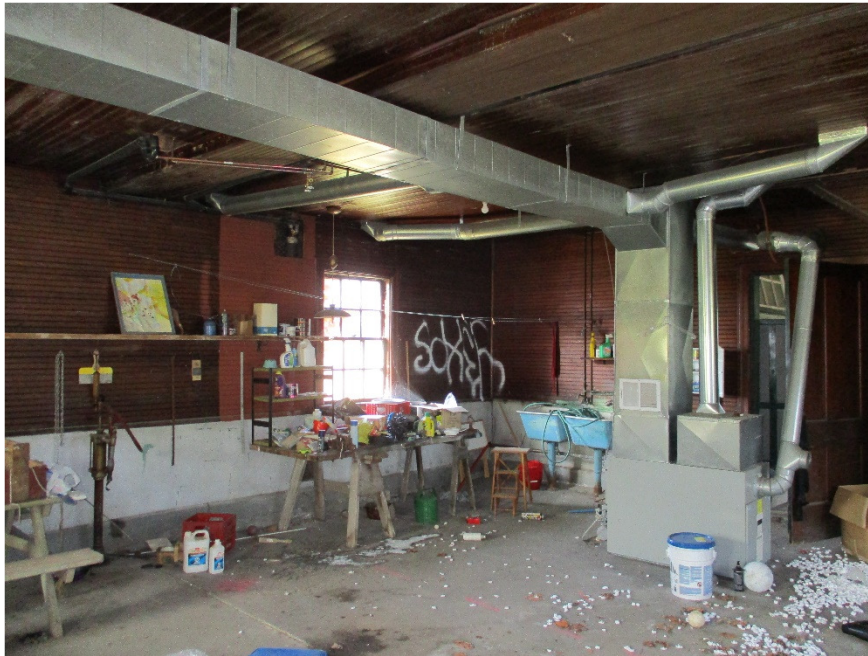
Interior of garage, note hand pump at left
