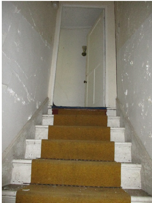
Stairs to apartment
