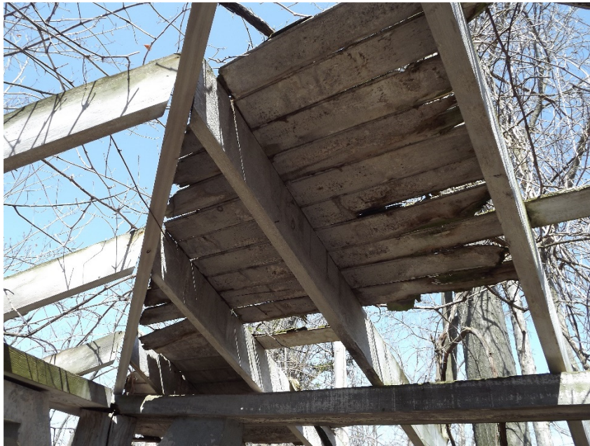
Remnant of roof sheathing, rafters, and plank beam, northwest corner
