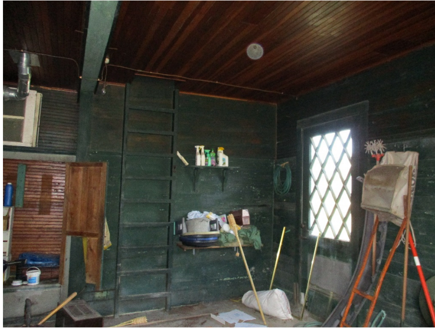
Interior of workshop, note ladder to hay loft
