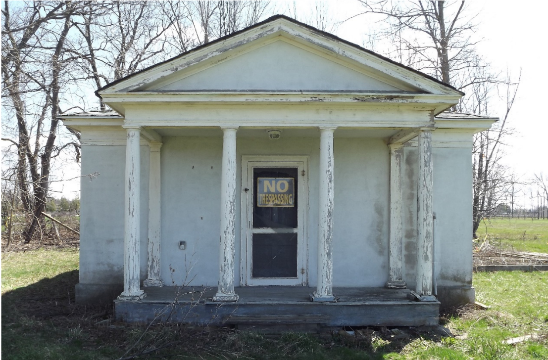
The Bath House West Elevation, April 2022
