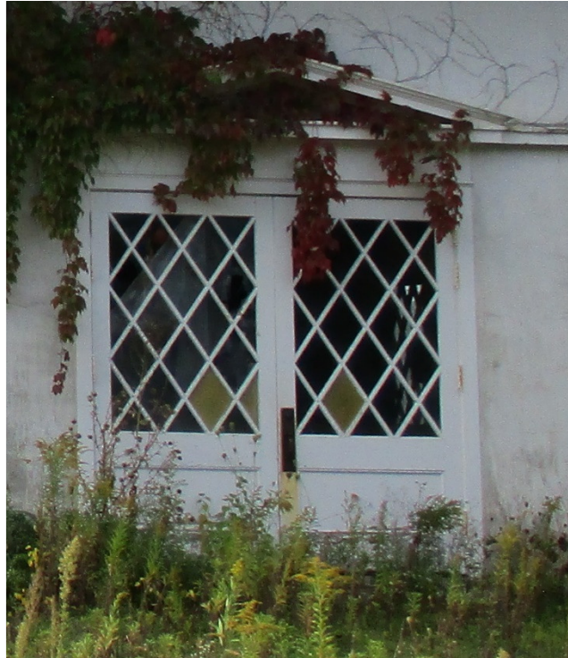
Drive doors to the workshop
