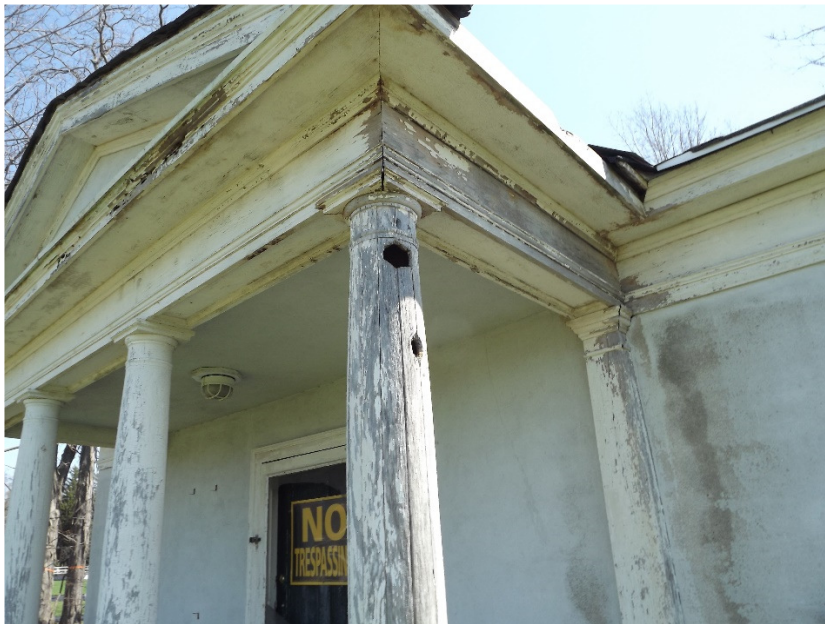
Porch floor and column bases requiring replacement
