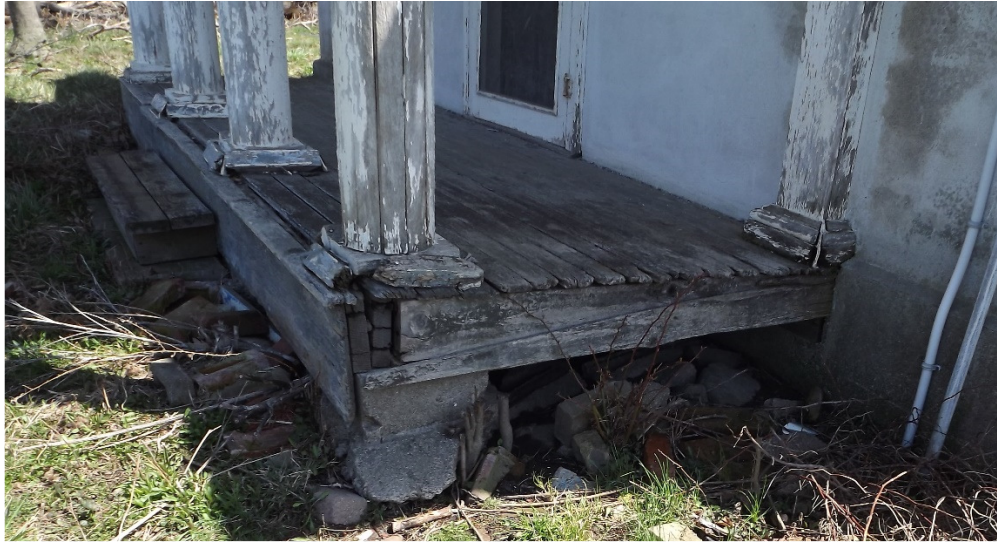
Porch floor and column bases requiring replacement
