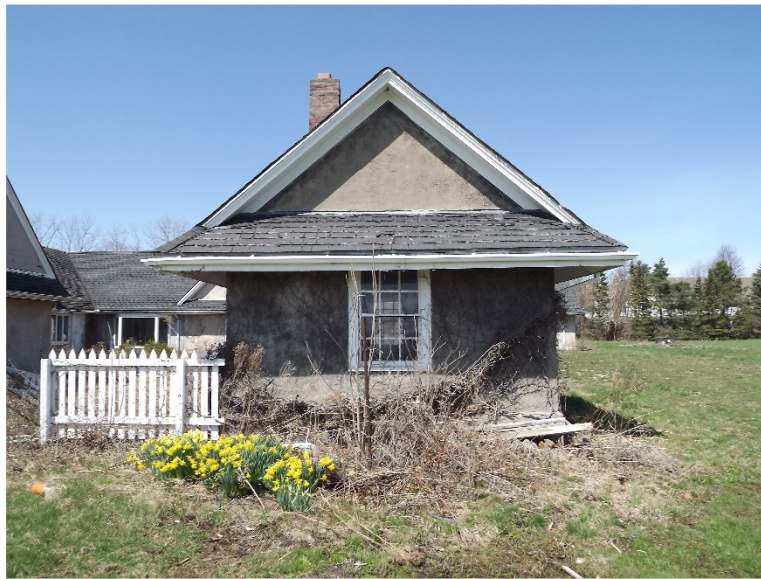
East elevation of Building B - Workshop
