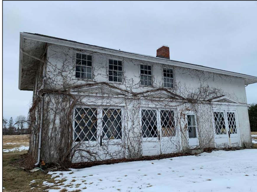
Figure 30 - The Carriage House, 200 John Street East, March 2023.
