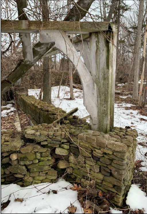
Figure 24 - Whistle Stop with wood bracket detail, March 2023.
