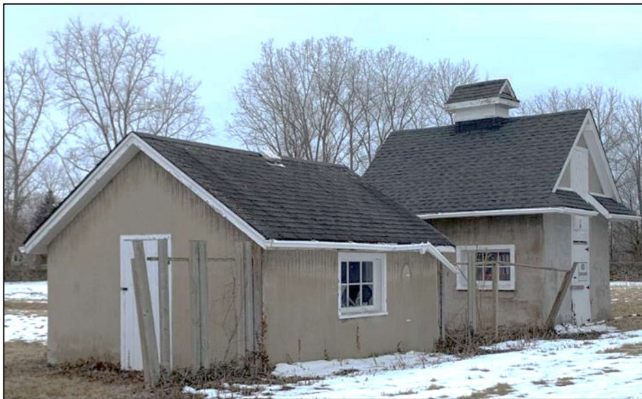
Figure 2 – Two Shed buildings, northeast elevation. March 2023.
