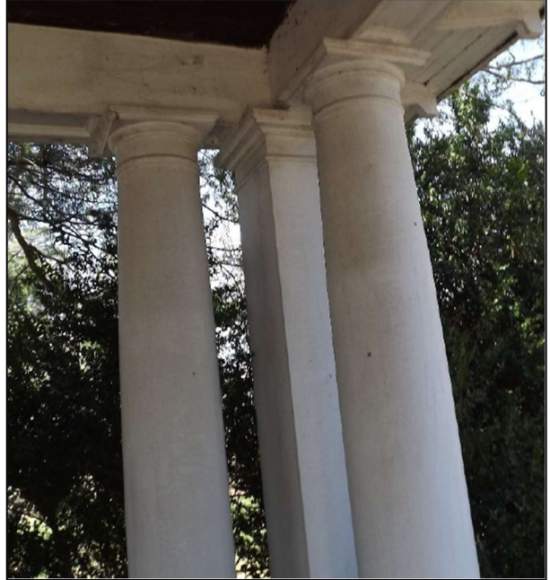
Figure 20 - Tea House with Tuscan-Style Columns, April 2022. Shoalts, Building Condition Assessment - The Tea Pavilion, 7.
