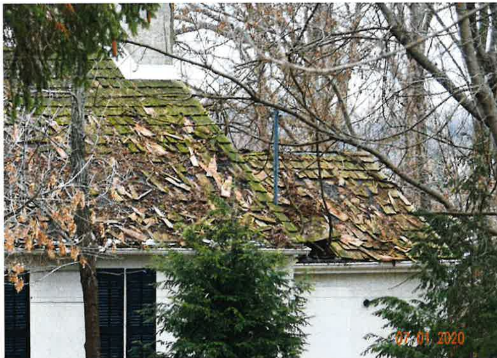
Figure 5: Cedar Roof on House and Addition
