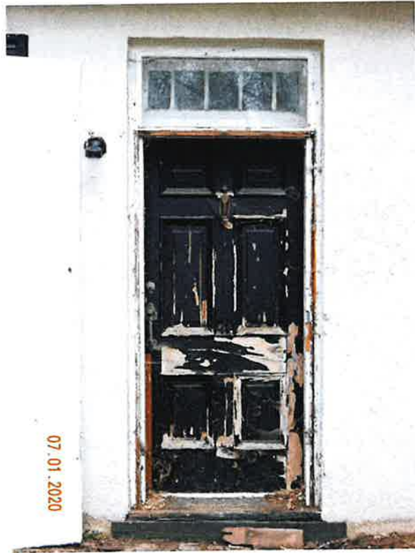
Figure 2: Entrance Door with 5-Light Transom
