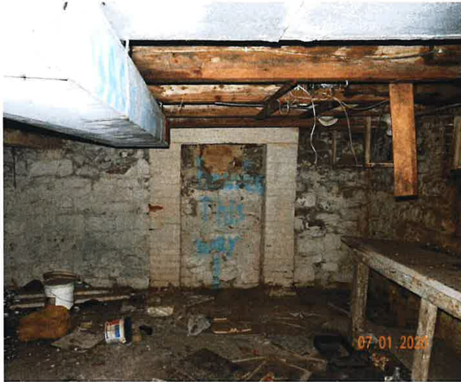
Figure 17: Basement Fireplace Foundation
