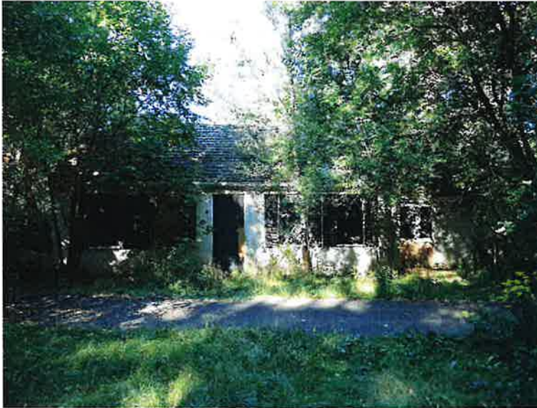
Southwest elevation, principal facade (ERA)
