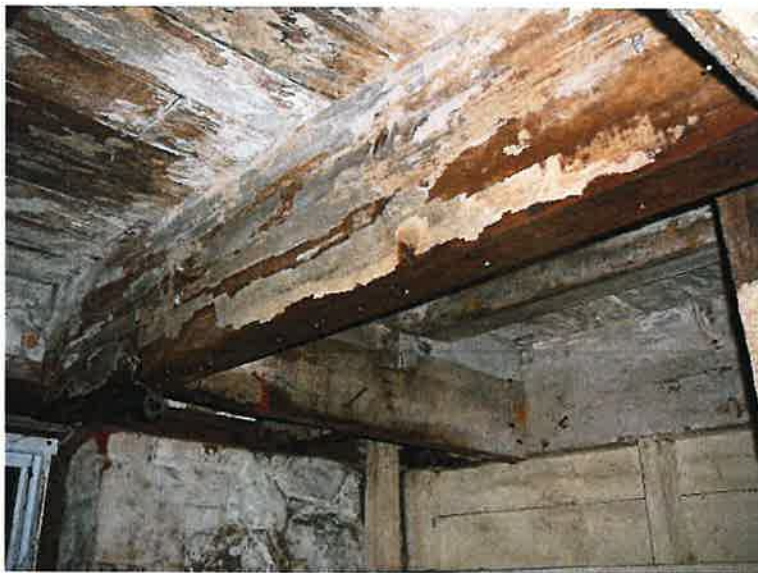
177 Byron ground floor joists. (ERA)
