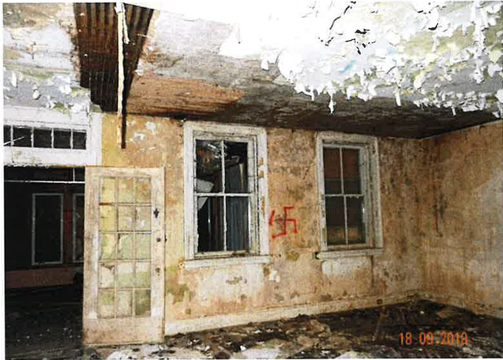
Figure 7: Interior Rear (North) Wall of Original House
