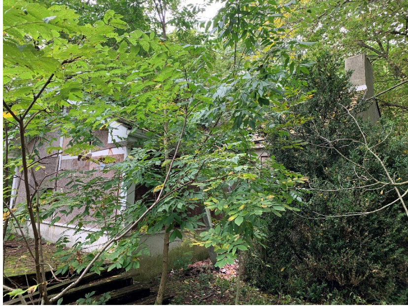
Figure 15: North elevation (rear) of dwelling with addition
