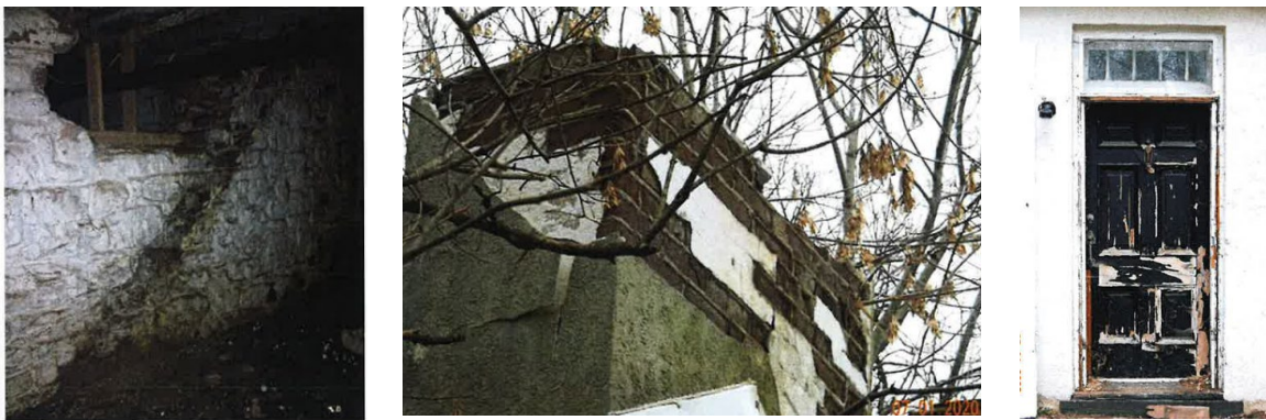
Figure 26 - 28: stone foundation located in basement, exterior chimney with brick, front door with original hardware (ERA, 2015)
