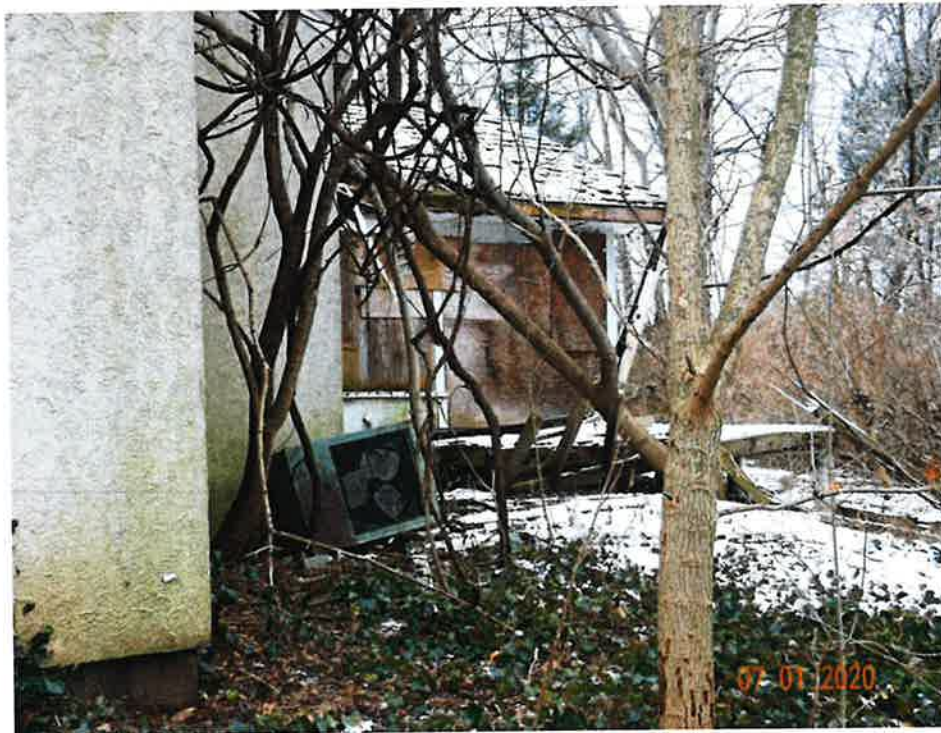
Figure 6: Rear Family Room Addition
