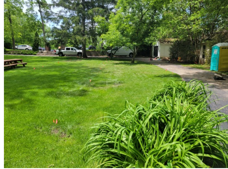
Image 10: View of site area after backfilling.
