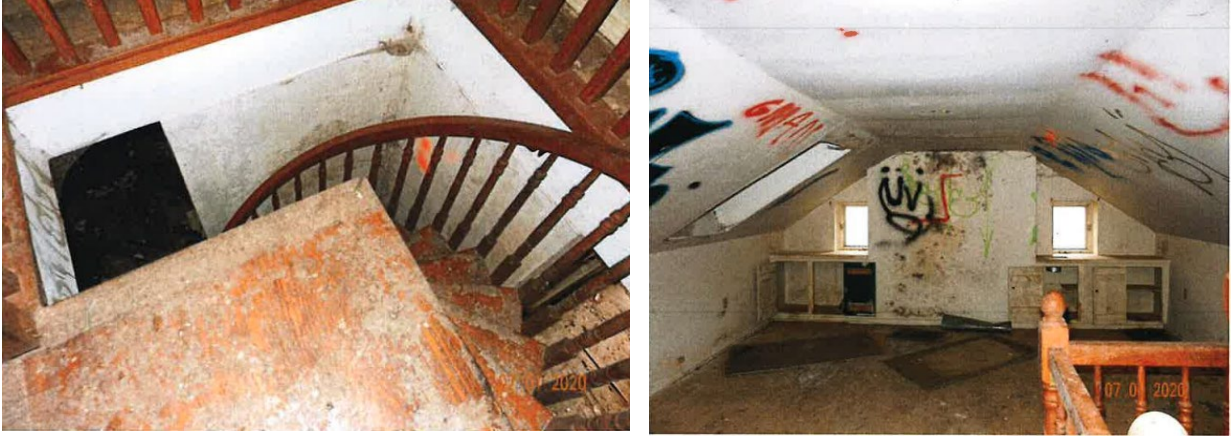
Figure 24 and 25: (left) spiral staircase leading to the attic, (right) attic (Wallace, 2021)
