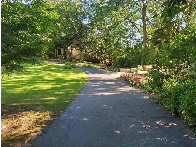
Image 1: View of disturbed asphalt driveway. Note sloped area on the right that has been stepped with patio stones.
