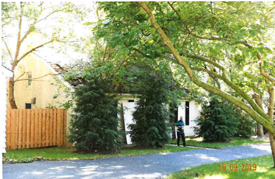
Figure 2: Facade with Fence to the West
