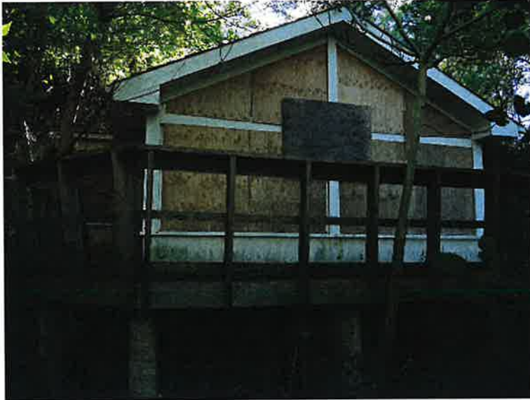
Northeast elevation, addition and deck (ERA)
