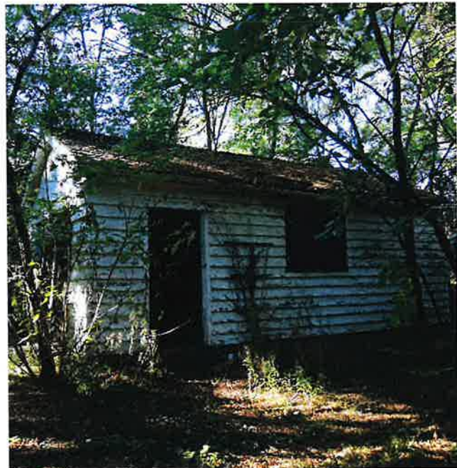
Detached garage west of house (ERA)
