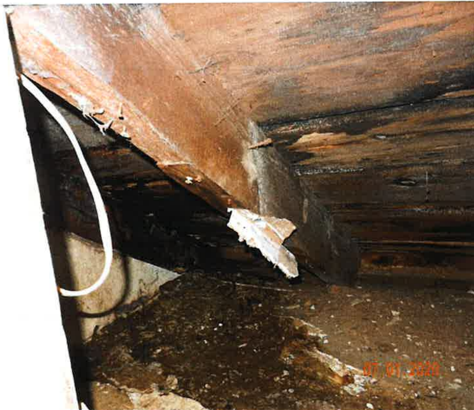
Figure11: Interior Roof Rafters
