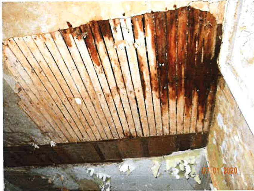
Figure 7: Ceiling with Modern Lath and In Floor Heating Unit
