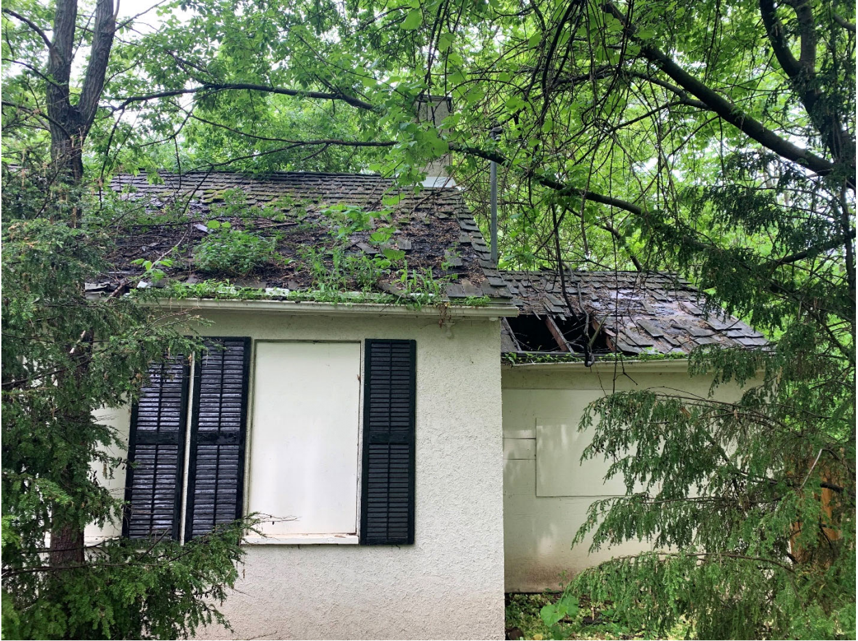
Figure 5 - Detail of dwelling on subject property, photo by Town Staff June 3, 2021
