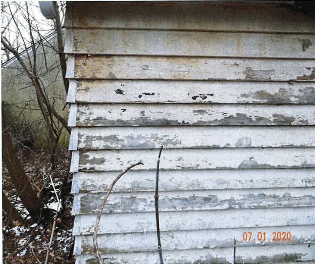
Figure 6: Garage West Wall at Corner
