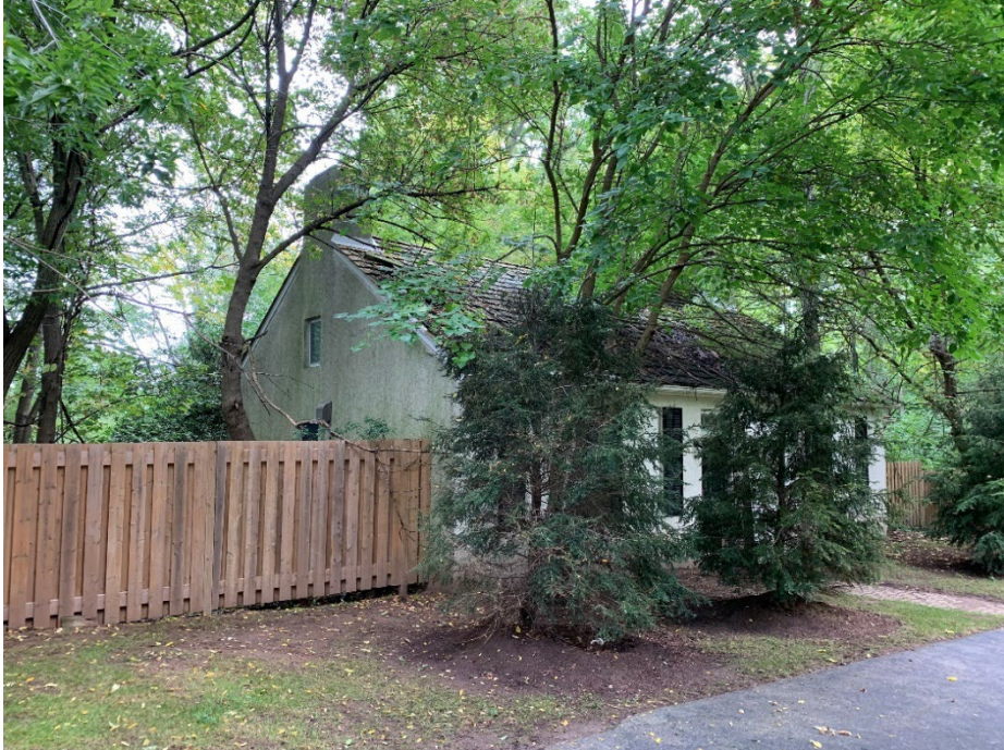
Figure 13: West elevation of dwelling
