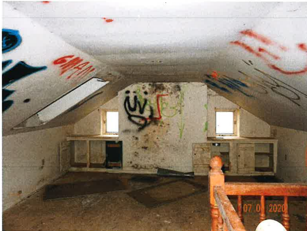
Figure 16: Attic with Newer Window Inserts at East End
