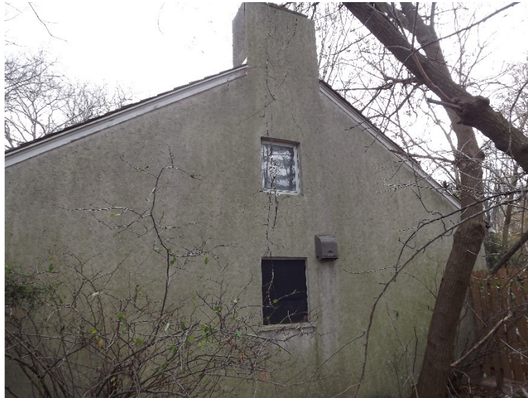
Two windows and an exhaust fan apparently through a chimney
