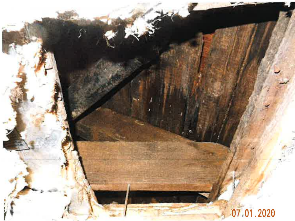
Figure 14: Roof Rafters and Structure
