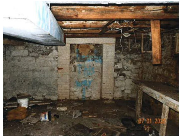
Figure 22 and 23: (left) staircase access as seen from basement, (right) basement with original fireplace foundation (Wallace, 2021)
