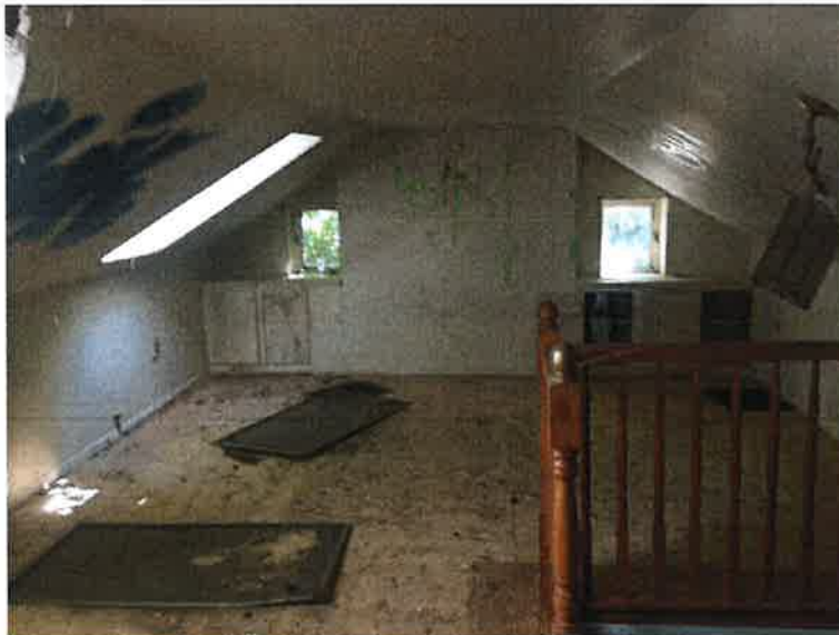
Attic, with new skylight and windows. (ERA)
