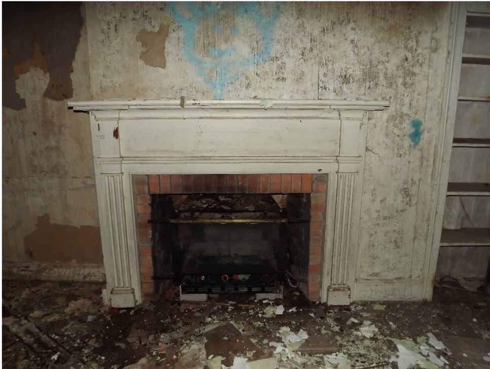
Fireplace with soldier course of bricks on a steel lintel
