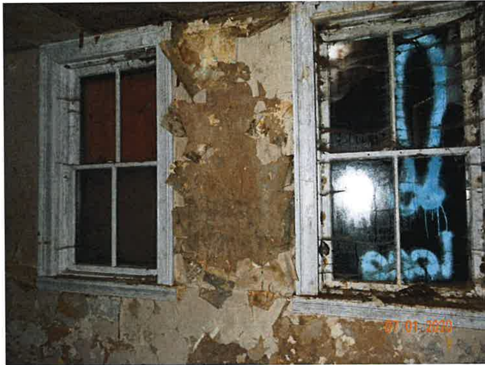
Figure 11: Interior South Wall
