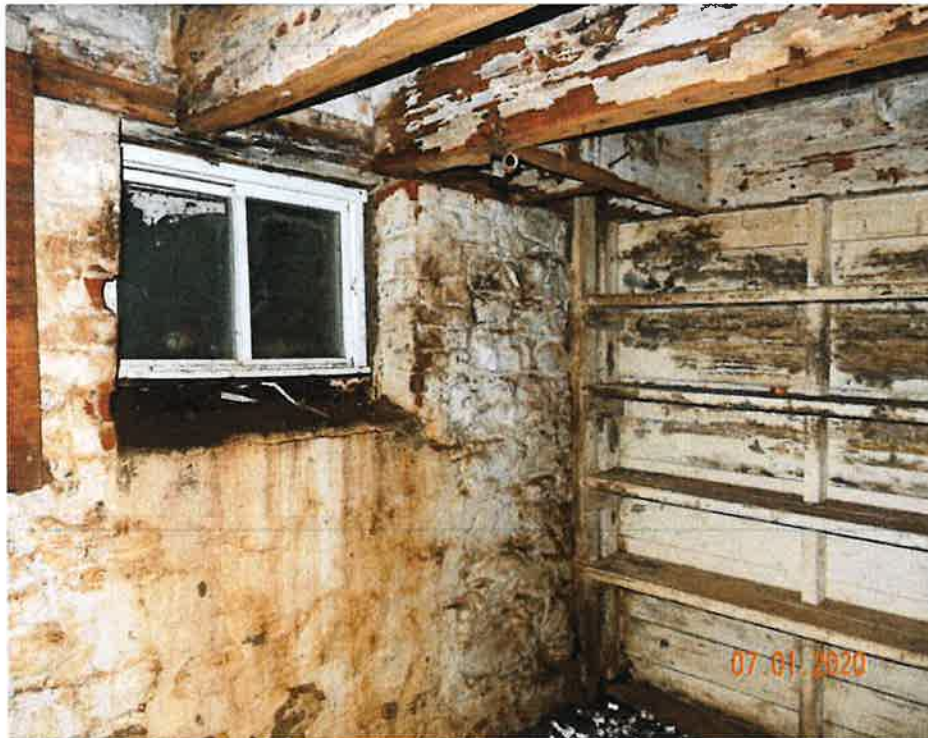
Figure 18: Basement Wall with Floor Joists
