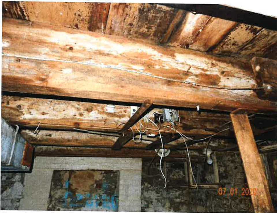
Figure 20: Basement Floor Joists and Floor Above
