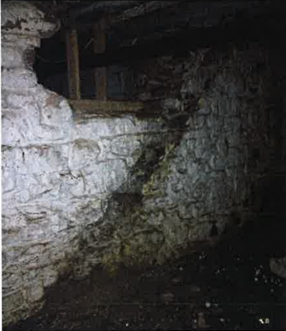
Basement, evidence of former stair. (ERA)
