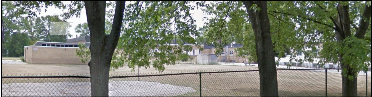
Image 10: Rear schoolyard showing the extensive later additions to Virgil Public School, clad in buff brick and projecting north into the lot. (Image Source: Google Streetview, 2012)
