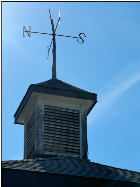
Image 4: Cupola / Bellcote of the 1872 one-room schoolhouse. The cupola is rectilinear in form, with a pyramidal/hipped roof and wooden louvers on the four sides. Note that the weathervane is a replica of the original. The original weathervane and bell have been relocated for display at Crossroads Public School in Virgil.
