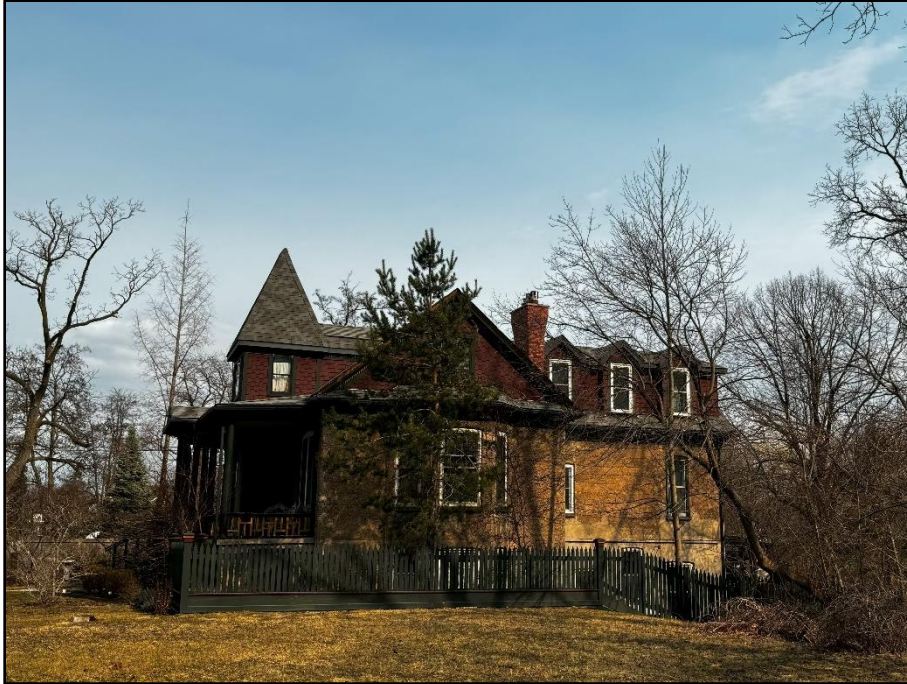
Image 3: South Elevation of Subject Property (Image taken on: February 28, 2024)
