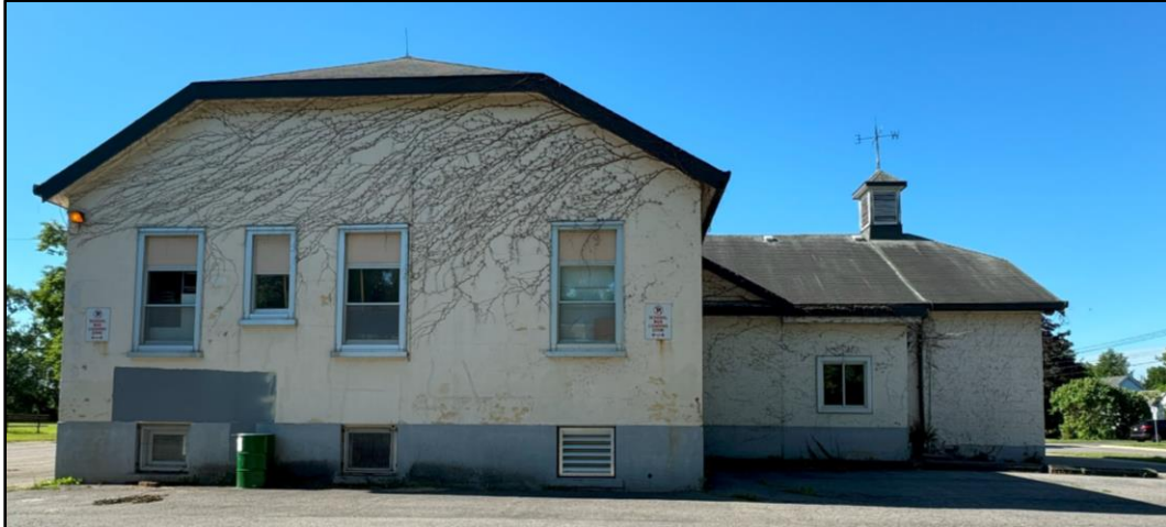
Image 7: West elevation of the 1872 one-room schoolhouse, showing the rectilinear addition that expanded across the rear of the 1872 building. The 20 th century addition has basement windows, and models the style of its opening and roof profile, albeit on a larger scale, from the 1872 design. (Image taken on: June 28, 2024)
