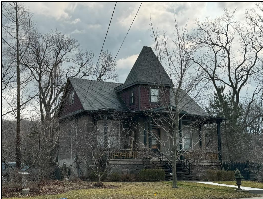
Image 4: Northwest Corner of Subject Property (Image taken on: February 28, 2024)
