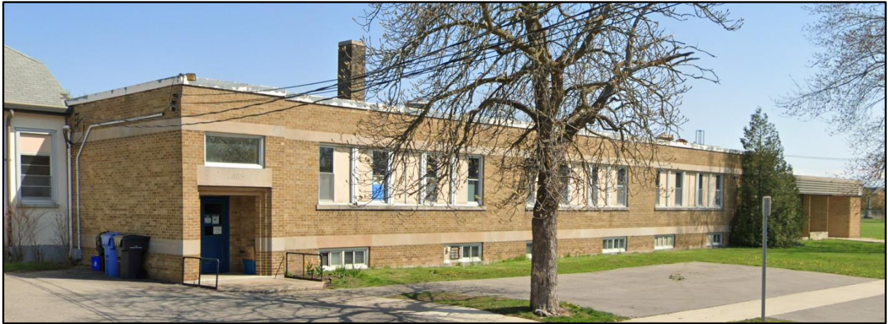
Image 12: Primary façade (south elevation) of the eastward expansion to Virgil Public School. The westernmost portion of this building projects forward, and includes a carved stone lintel over the portal that reads 'Girls', replacing an earlier entrance with the same functionality. Horizontal stone lintels and stringcourses emphasize the rectilinearity of the buff brick clad building. This image also illustrates the narrow depth of the setback from the sidewalk and street that was characteristic of the relationship between the original 1872 schoolhouse situated close to the public realm.
