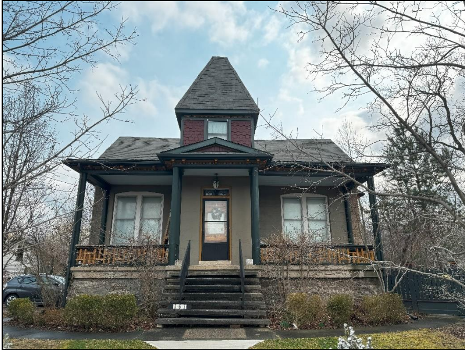
Image 1: West Elevation (façade) of Subject Property (Image taken on: February 28, 2024)
