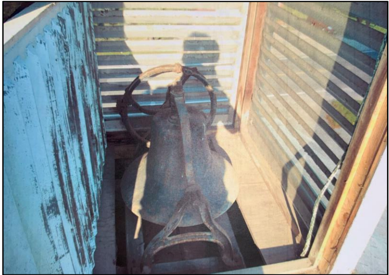
Image 14: View into the bellcote located on the roof of the original 1872 school building. This bell has been relocated and remains on display at Crossroads Public School.
