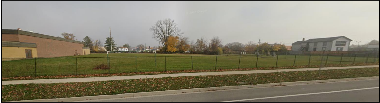
Image 13: East elevation illustrating the infill between earlier 20 th century buff brick clad expansions, with a taller gymnasium connecting the south and north arms of the school. This image also illustrates the expansion of the schoolyard to the east of the school building into the later 20 th century. A sidewalk extends along the south perimeter of the lot, and the schoolyard is demarcated by a chain link fence.
