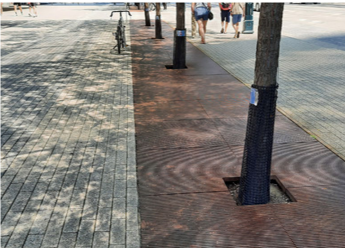
Trees in hard paving with connected soil volumes
