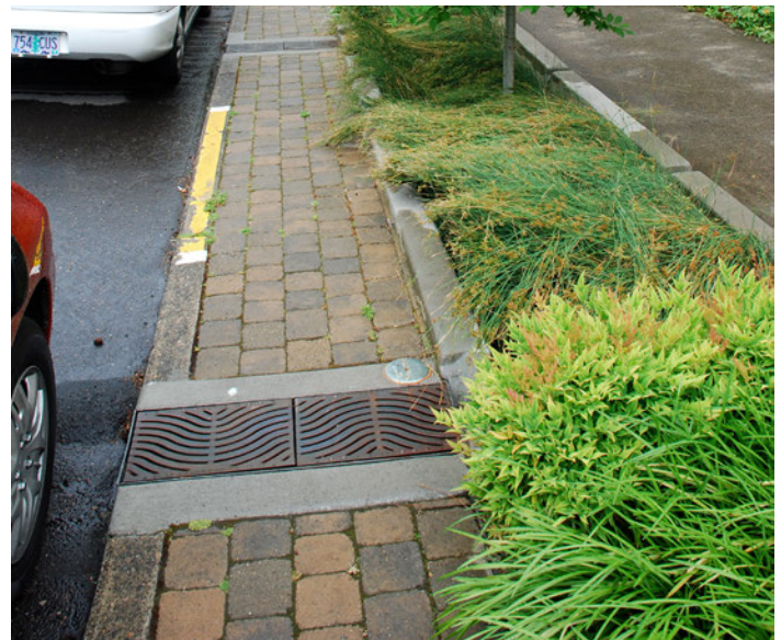
Bioretention planters for stormwater management, Portland OR
